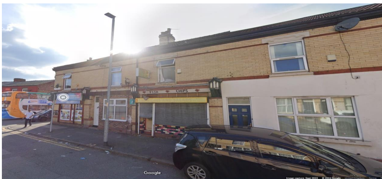
Numerous precedents of corner shop and mid terrace retail conversions exist in the local area e.g. Mathews Lane/ Stovell Avenue
