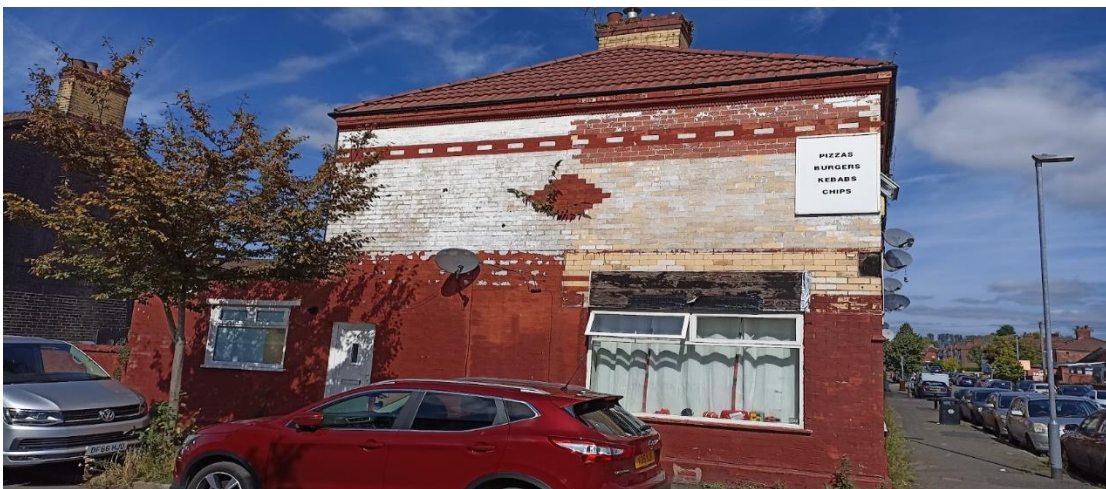
No significant alteration on the side elevation, aside from the installation of new signage and the painting of the external render, alongside front window replacement. Due to the premises' historical use as a hot food takeaway, there are already separate entrances for the retail unit (via Hemmons Road) and the residential unit (via Longdon Road). These distinct access points ensure that the resident occupying the upstairs flat will not be affected by the retail activities on the ground floor, maintaining privacy and minimizing disruption
