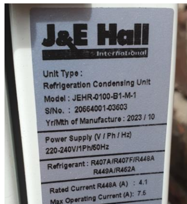
Figure 11 Spec of the condenser unit
