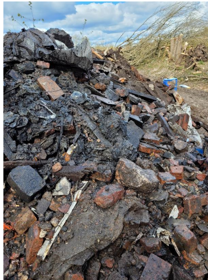
Figure 3. Example area coverage by visually hazardous materials that would be supportive of ceasing the excavation
