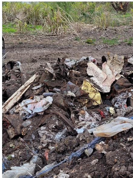
Figure 5. Example area coverage by visually hazardous materials that would not be supportive of ceasing the excavation
