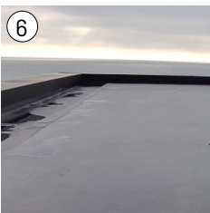
Single ply membrane roof
