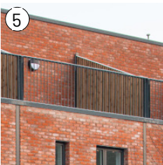
Steel balcony balustrade
