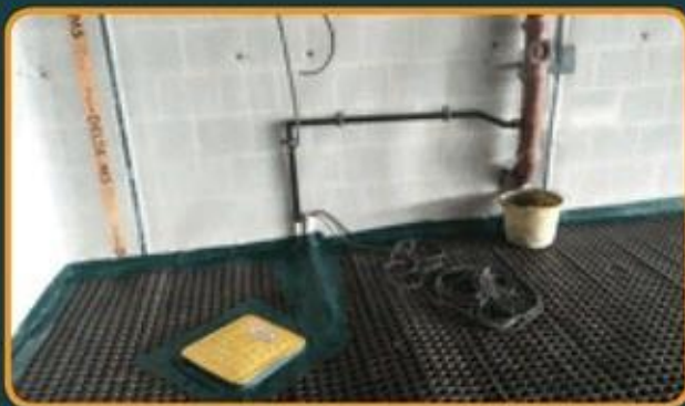
The pumping system is installed in a sump chamber, connected to the drainage channels.
