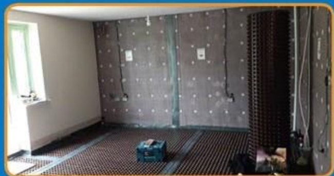
8mm wall membrane and 20mm floor membranes, joints taped and overtaped.
