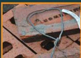
Cavity Wall Tie Repair
