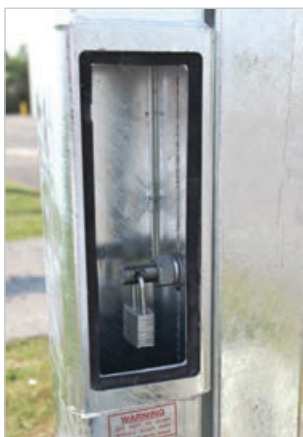
Tilt-down columns have the facility to be padlocked internally
