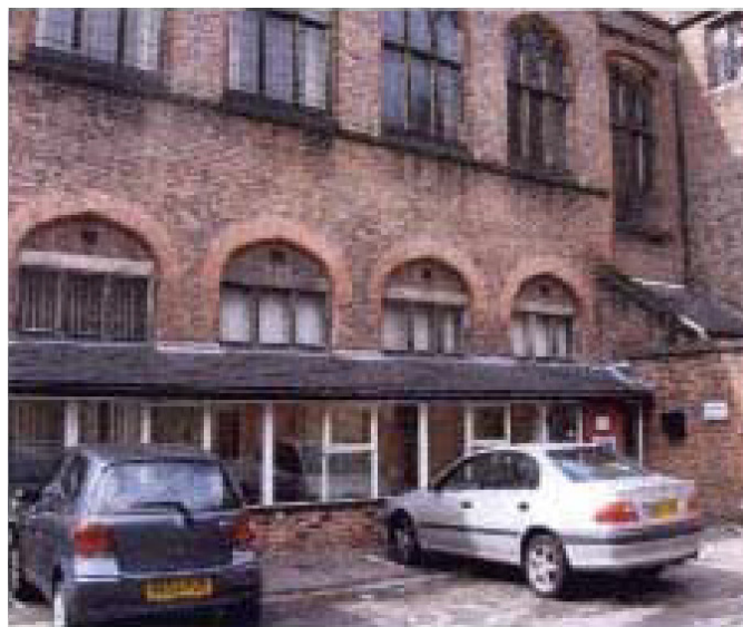
Fig.3: part-glazed corridor on east side of 1870s wing, rebuilt in 1971 and demolition in 2009
