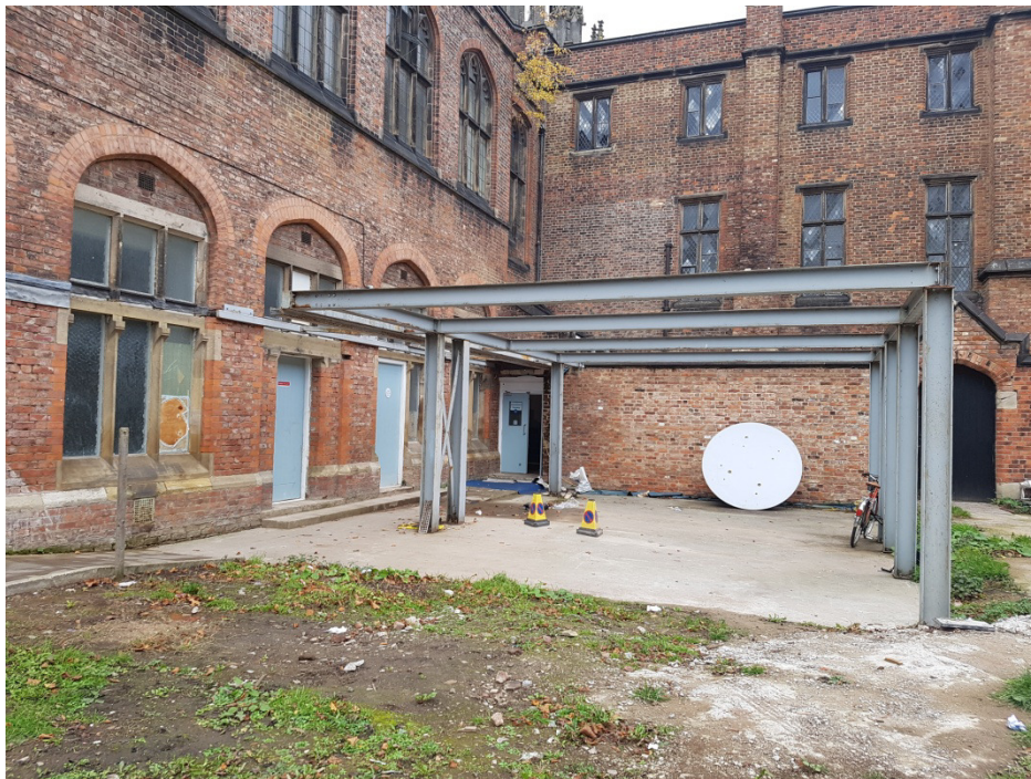
Fig.4: 2019 existing steel frame erected based on 2008 planning approval
