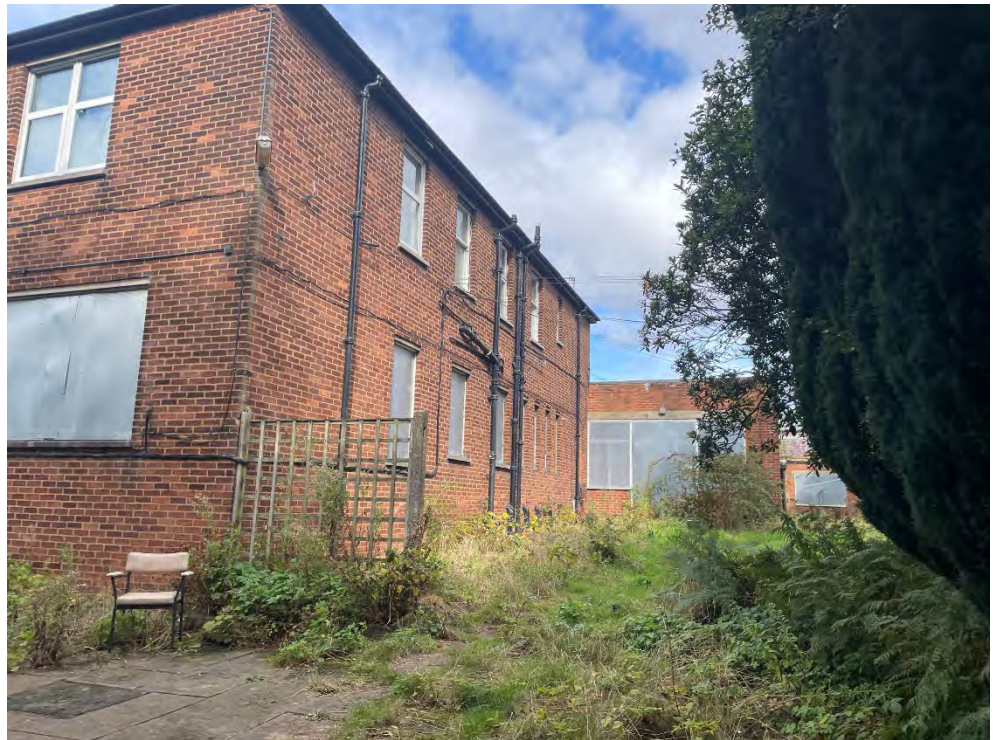
Plate 4 View of an extension at the northern elevation of the former convent building
