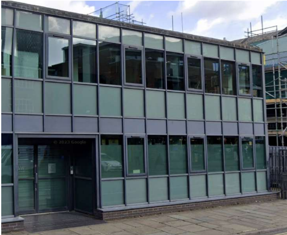
Existing Photo - Liverpool Road Facade
