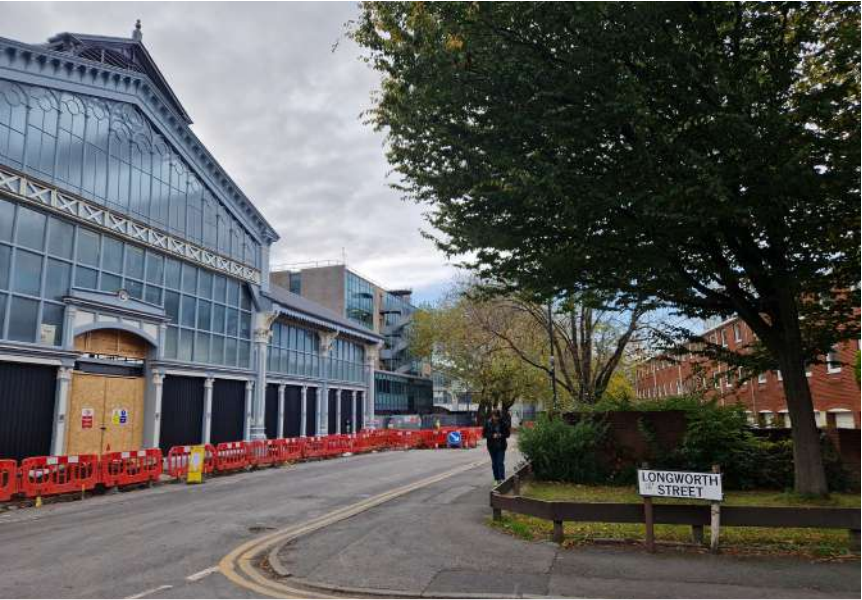
View from Tonman Street (north-east)
