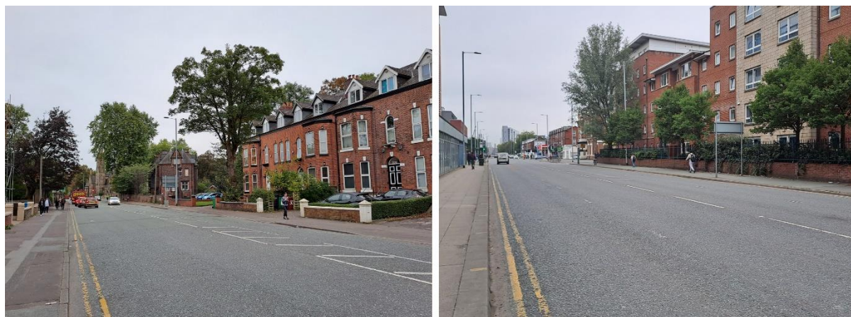
Figure G: Upper Brook Street around the Junction with Hathersage Road
