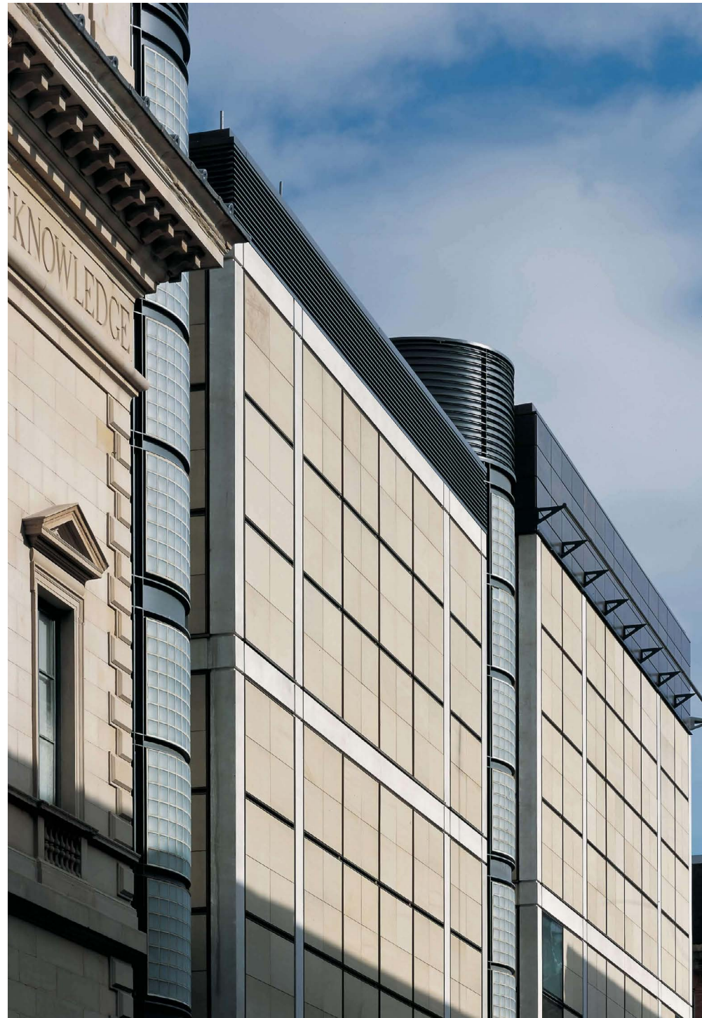
Figure 5 2002 Extension, Exterior © Hopkins Architects 9
