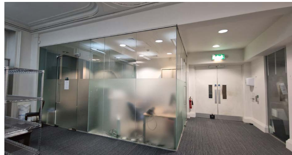
Figure 20 Photograph showing modern glazed partitions and screens to be removed
