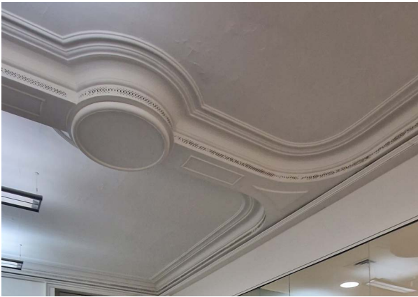
Figure 28 Photograph showing high level metal grilles in B02-B2-003
