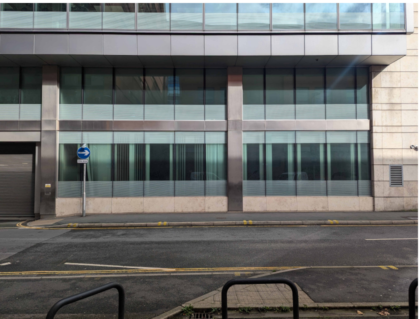
Photo of L01 South facade as existing
