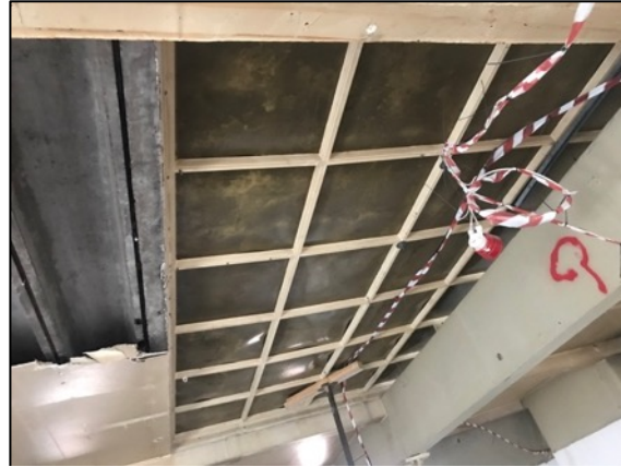
24. Later 20 th century former skylight of no heritage significance. Proposed to be removed.
