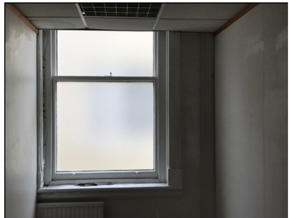
43. Single one over one sliding sash window example.
