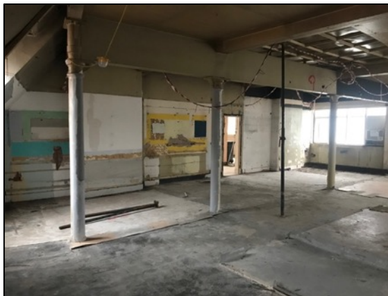
21. Series of cast iron columns (2).
