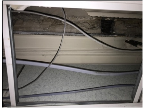
42. Partial survival of original plaster run decorative cornice.
