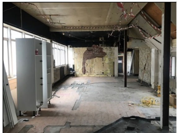
16. General view across the floorplate of the early 20 th century warehouse, looking east.
