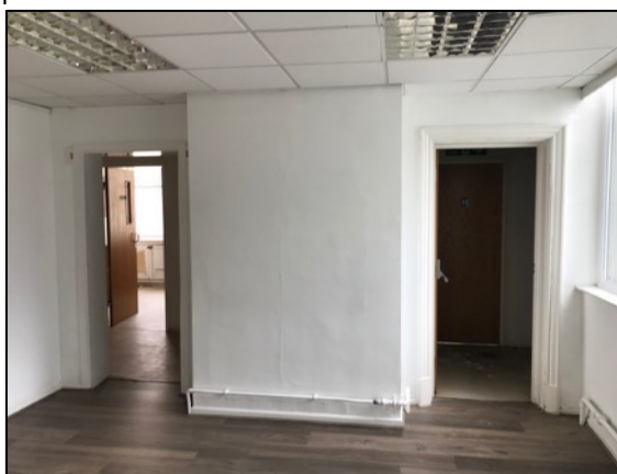
37. Cast iron columns enclosed within plasterboard.
