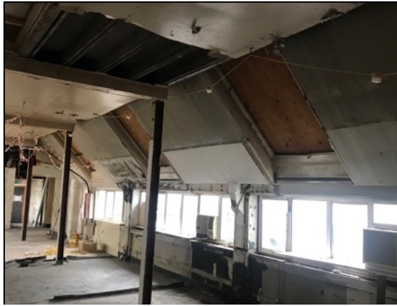
17. Three former timber framed skylights to the Mansard roof of the early 20 th century warehouse. Proposed to be concealed and retained.
