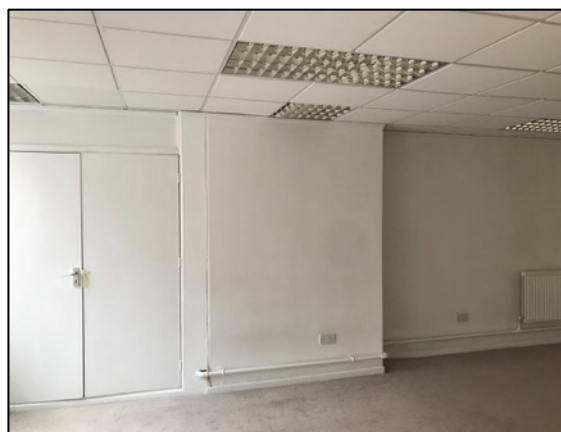
38. Original masonry chimneybreast retained.
