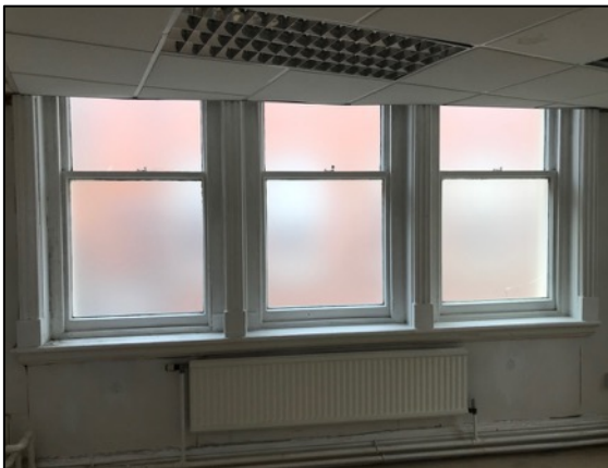
43. Original mid-19 th century one over one sliding sash windows to older section of floor plate.
