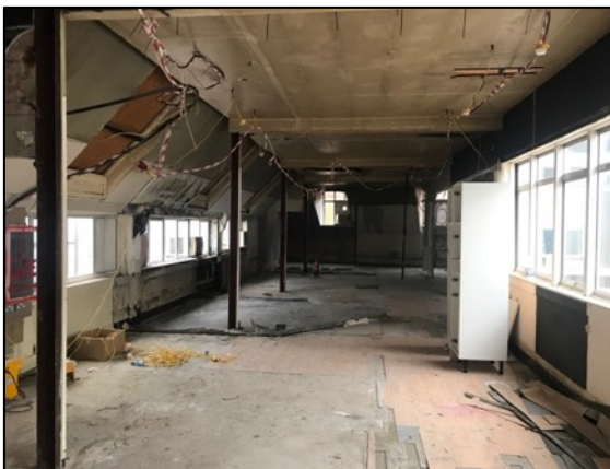
15. General view across the floorplate of the early 20 th century warehouse, looking west.
