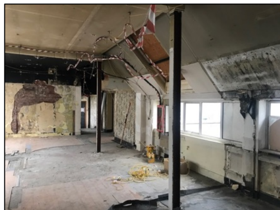
28. Later 20 th century steel structural columns of no heritage interest.
