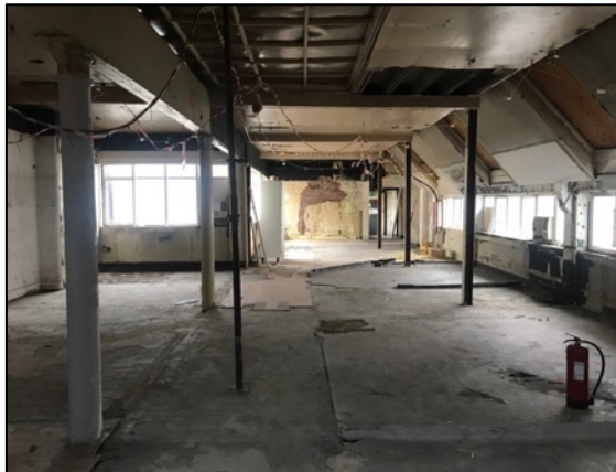
19. General view across the floorplate of the warehouse with cast iron columns to the left.
