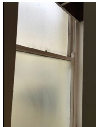
46. Example of slightly later replacement timber framed sliding sash window with horns.
