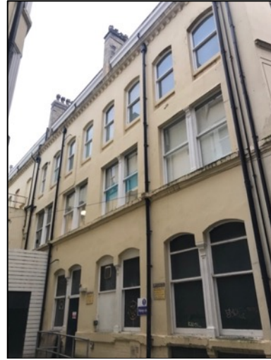
6. The mid- to late- 19 th century former grocery store and offices forming the northern portion of the site and containing part of Suites 2F and 3F.
