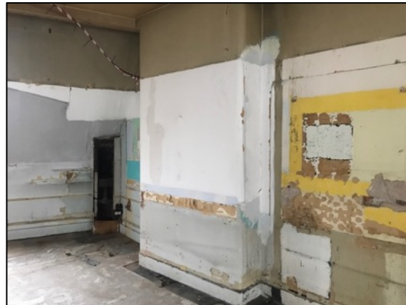
26. Detail of retained chimneybreast (2).
