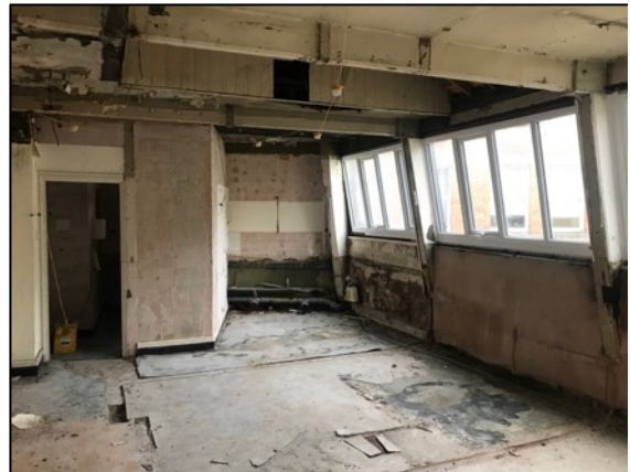
10. Westernmost portion of the former grocery store and offices.
