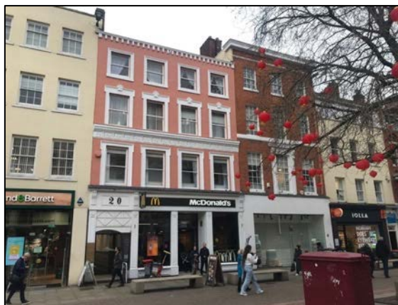
1. No. 20 St Anns Square, east elevation facing St Anns Square. Note the Greek Revival scheme of decoration to the upper floors, indicating an early 19 th century date for the original townhouse.
