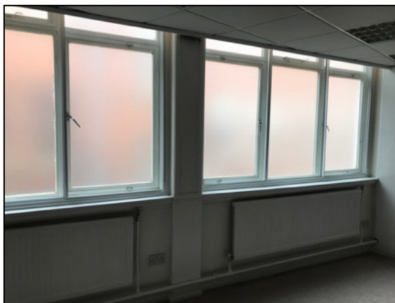
35. Structural elements enclosed between windows to former warehouse building.
