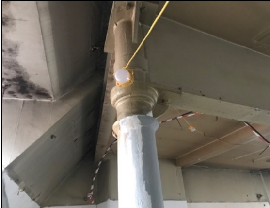
23. Detail of truncated column capital to westernmost column adjacent to Barton Square.
