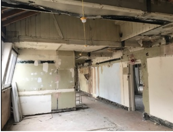
7. Interior of the former grocery store and offices, forming the northern section of the floorplate of Suite 3F, looking east. Note the timber boarding which forms part of the skylight above.
