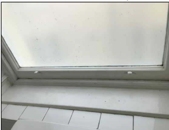
45. Detail of original sash pulls.
