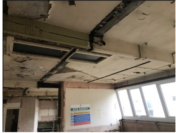
12. Detail of timber ceiling beam. Note the traditional chamfer and stop detail.
