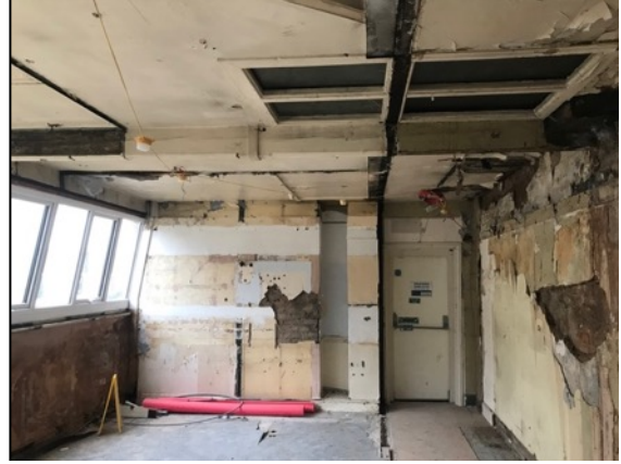
8. General view of the easternmost section of the former grocery store and offices, looking eastwards towards the emergency fire escape.
