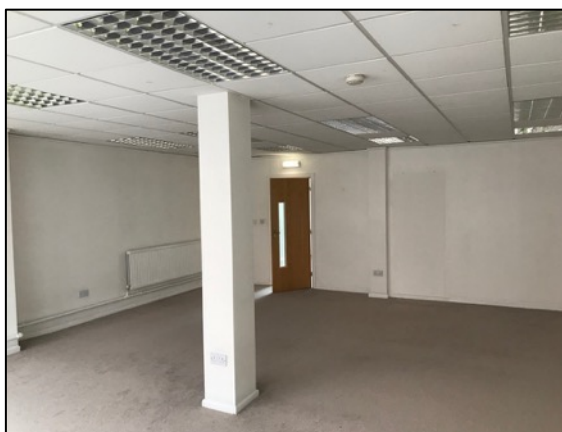
37. Cast iron columns enclosed within plasterboard.
