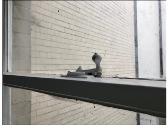
30. Detail of original sash catch ironmongery to timber framed sliding sashes.
