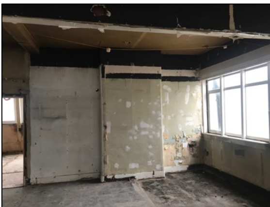
27. Detail of retained chimneybreast (3).
