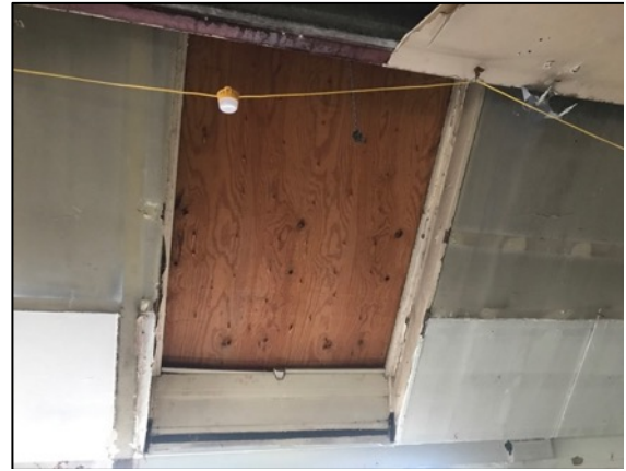
18. Detail of former timber framed skylight, closed during subsequent re-roofing works. Proposed to be concealed and retained.
