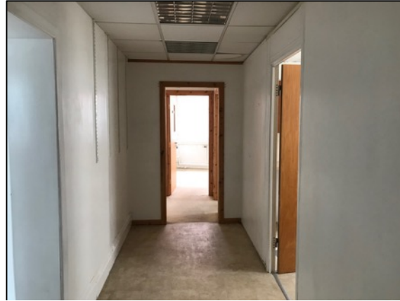
48. Corridor within former grocery store and offices, all visible elements modern.
