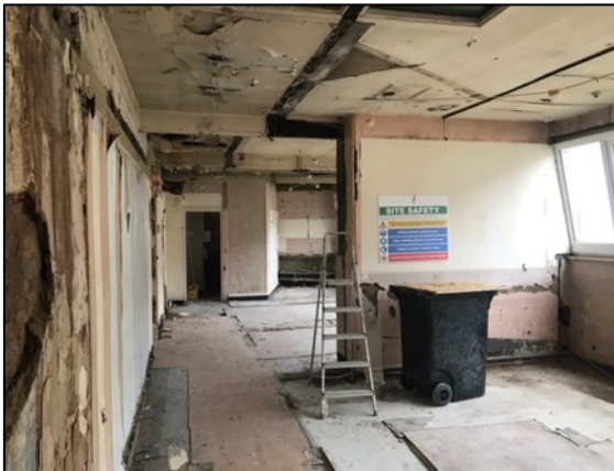
9. View looking westwards across the floor plate of the former grocery store and offices.
