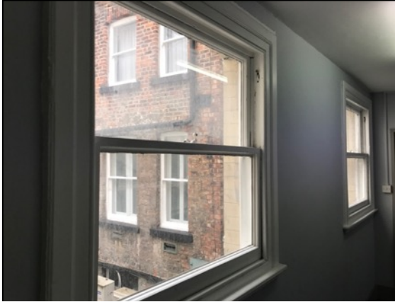
29. Pair of original mid-19 th century one over one timber framed sliding sash windows to corridor.
