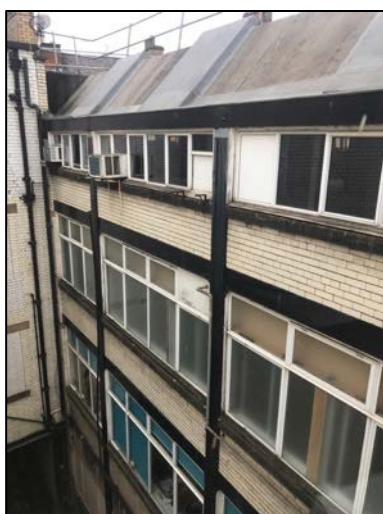
3. South elevation of the early 20 th century warehouse to the rear of 20 St Anns Square, containing part of Suite 3F.
