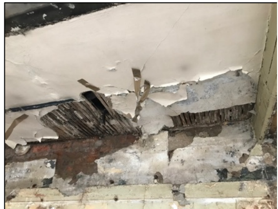
14. Retained section of lath and plaster ceiling (2).
