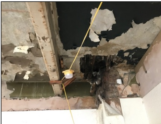
13. Retained section of lath and plaster ceiling (1).
