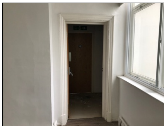
40. Original door frame and surround into former grocery store and offices.
