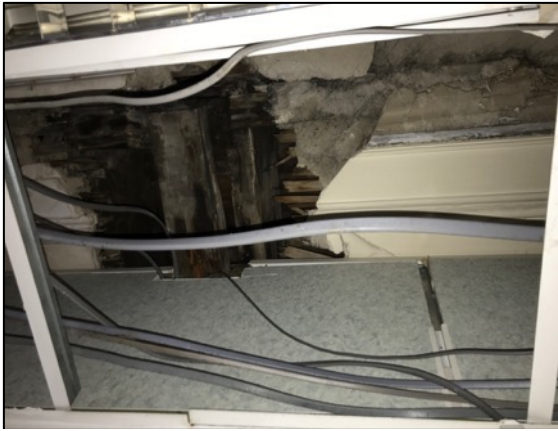
41. Partial survival of original lath and plaster ceilings within former grocery store.
