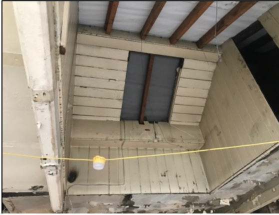
11. Timber framed former skylight within the former grocery store and offices. Proposed to be concealed and retained.
