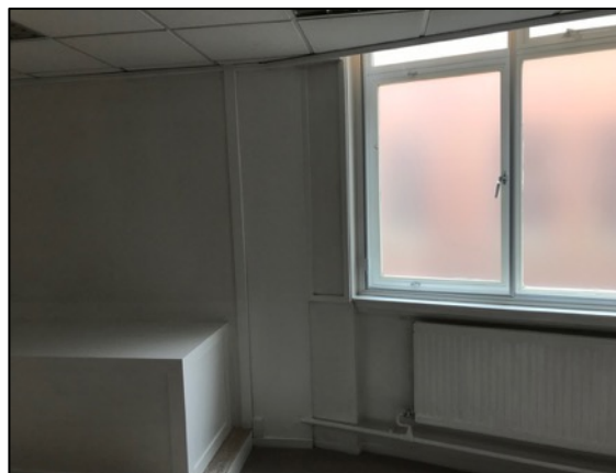
36. Structural element enclosure, assumed to be early steel frame or reinforced concrete frame.
