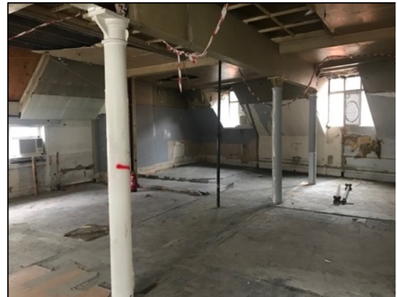
20. Series of three cast iron columns (1).
