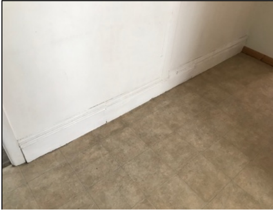
47. Typical surviving original section of timber skirting.
