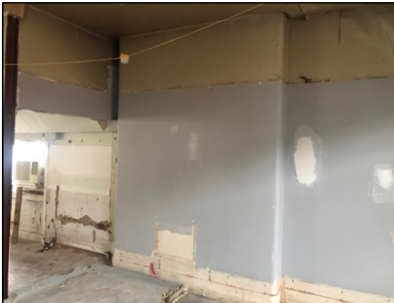
25. Detail of retained chimneybreast (1).
