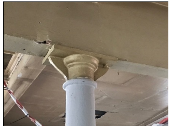
22. Detail of typical cast iron column capital.
