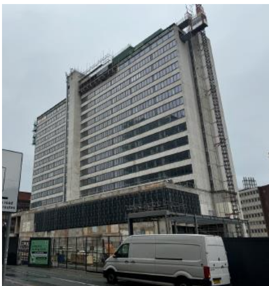
Present view of site from Deansgate
