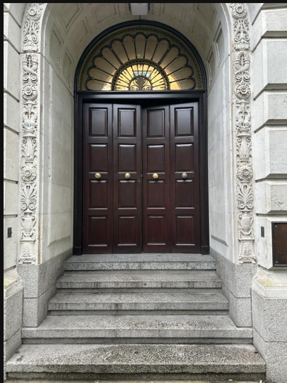
Existing fire doors with bifold outer doors closed
