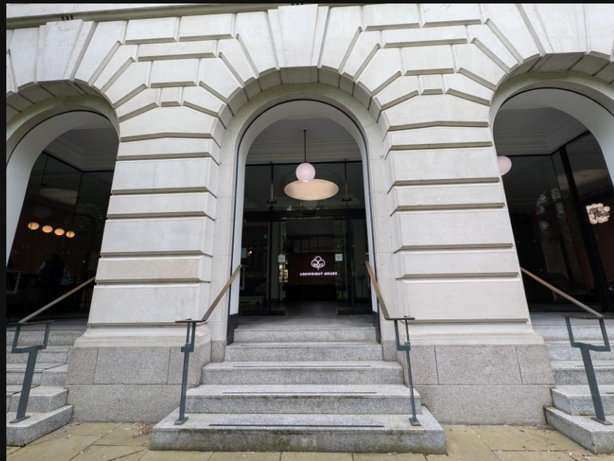
Existing main entrance 3 archways
