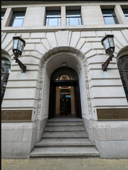
Existing fire exit with gas lamps & signage
