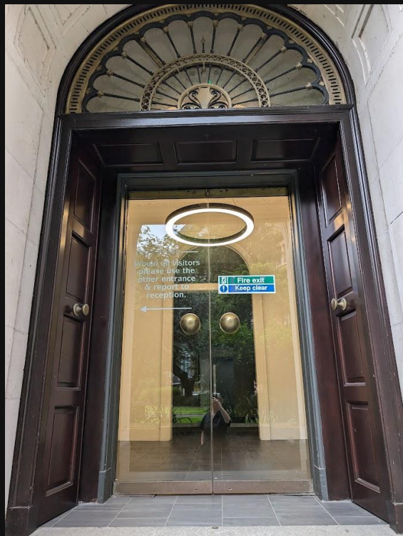
Existing fire doors with bifold outer doors open and glass inner doors
