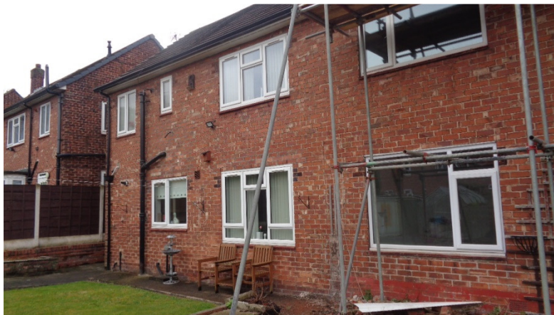
Adjoining Elevation of Application Property.
