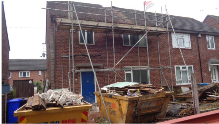
Front Elevation to Application Property.
