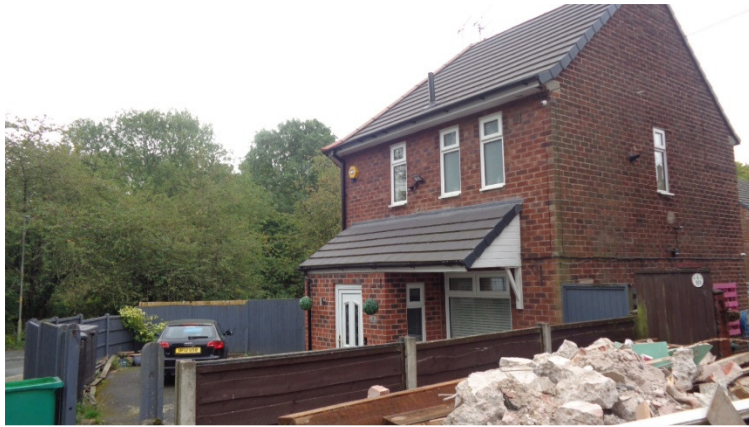
Adjoining Properties to Application Property.
