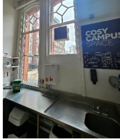
Board to window to be removed in G.005
