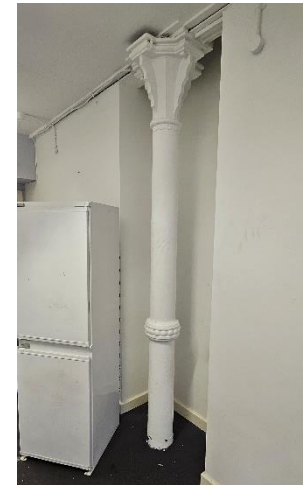
Existing ornate columns in basement B. 004
