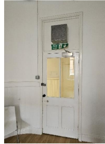
Existing doors to be retained. Black out film to door in G.006b
