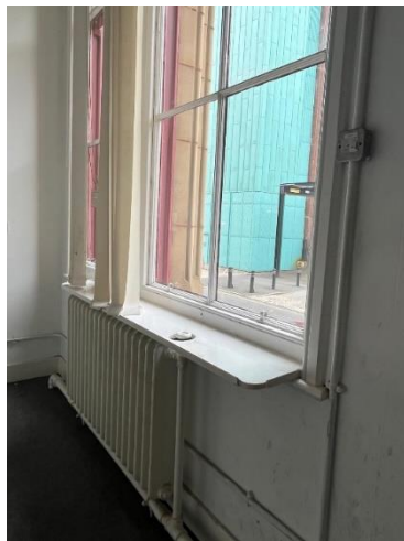
Existing cill and blinds at window in G.003 to be removed
