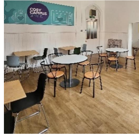
Existing vinyl to be removed in G.006
