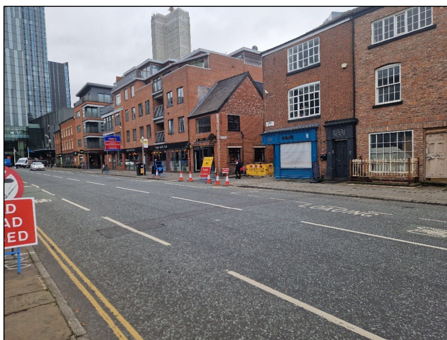
Image 2.2 Liverpool Road looking East
