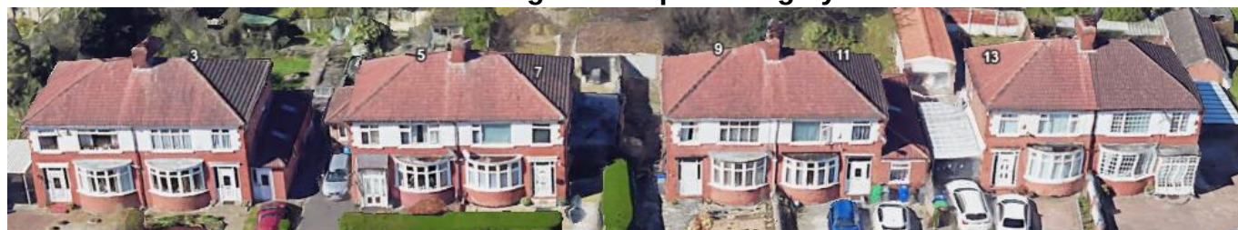
View of front-facing roof slopes along Lynton Drive
