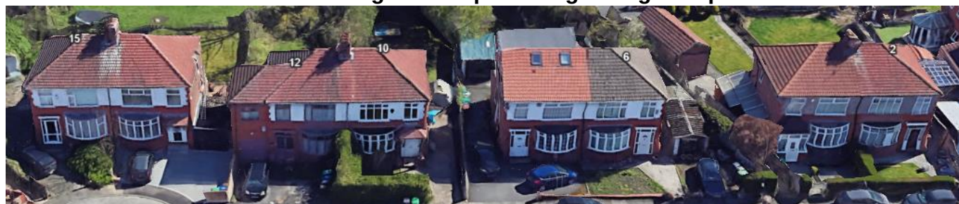
View of front-facing roof slopes along Lynton Drive
