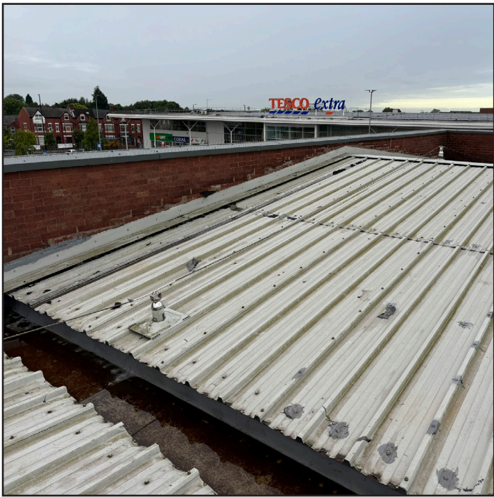
Figure 9 - Parapet to Roof Junction
