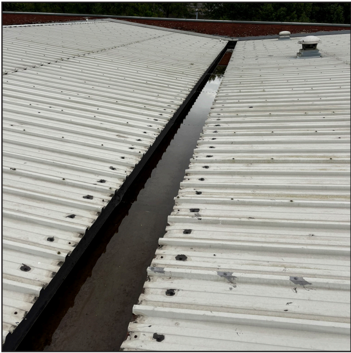
Figure 10 - Example of Existing Valley Gutter at Gorton Market.
