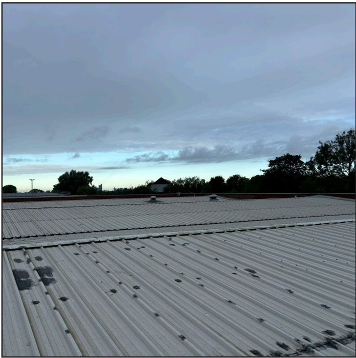
Figure 8 - Existing Roof finish at Gorton Market
