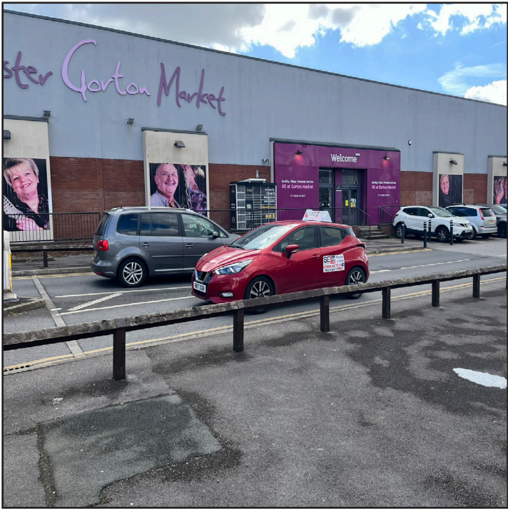
Figure 4 - Main Entrance into Gorton Market (West Elevation)
