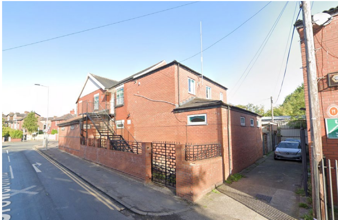
Rear/ Side of Building with rear access
