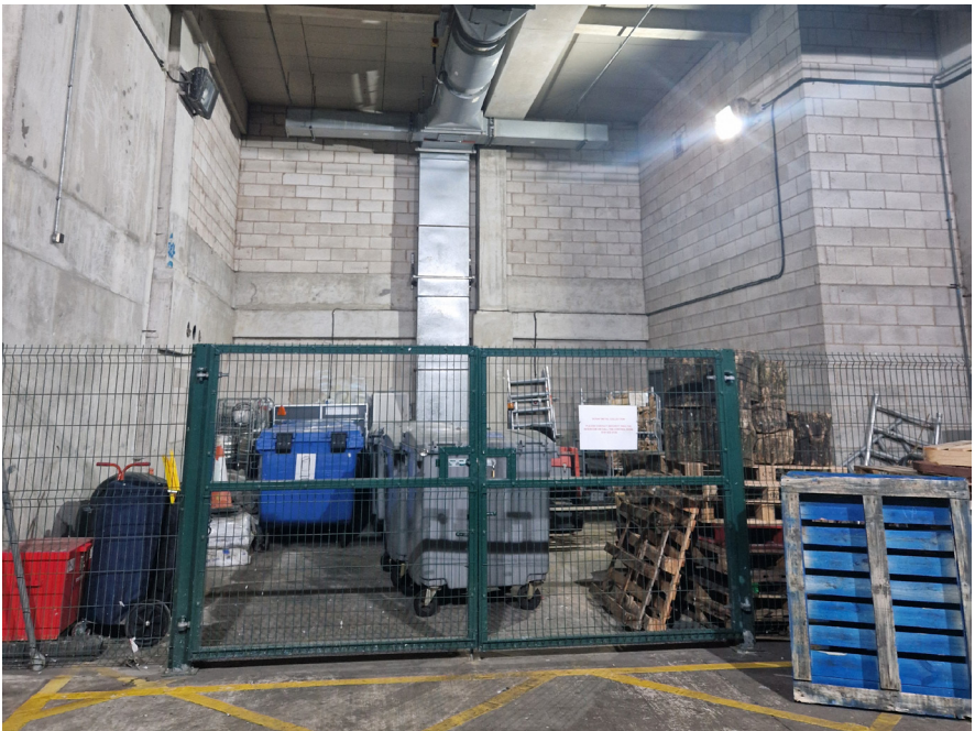
PLANT AREA OPPOSITE PROPOSED WORKS
