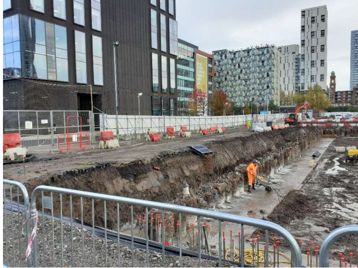
Plate 54: Wednesday 16 th November 2022. Overview of foundation piles.
