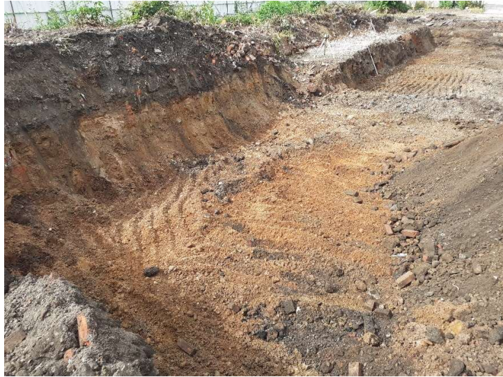
Plate 42: Tuesday 6 th September 2022. Excavated made ground.
