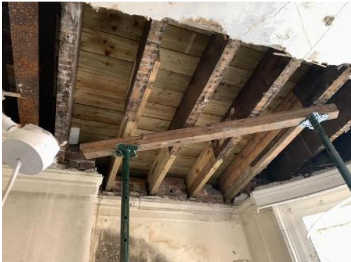
Above: Upper ground floor room with front bay extension. North west corner of ceiling.
