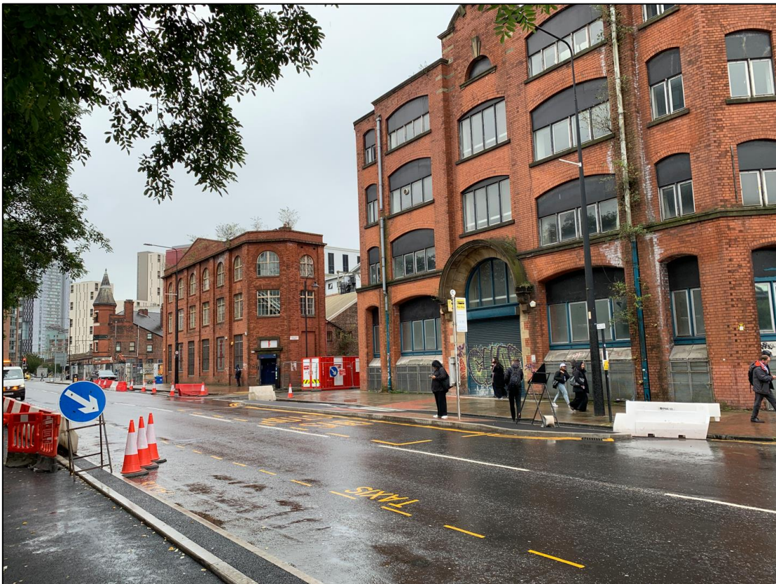
Figure 2.6 – South-East Facing View of Whitworth Street West and the Site
