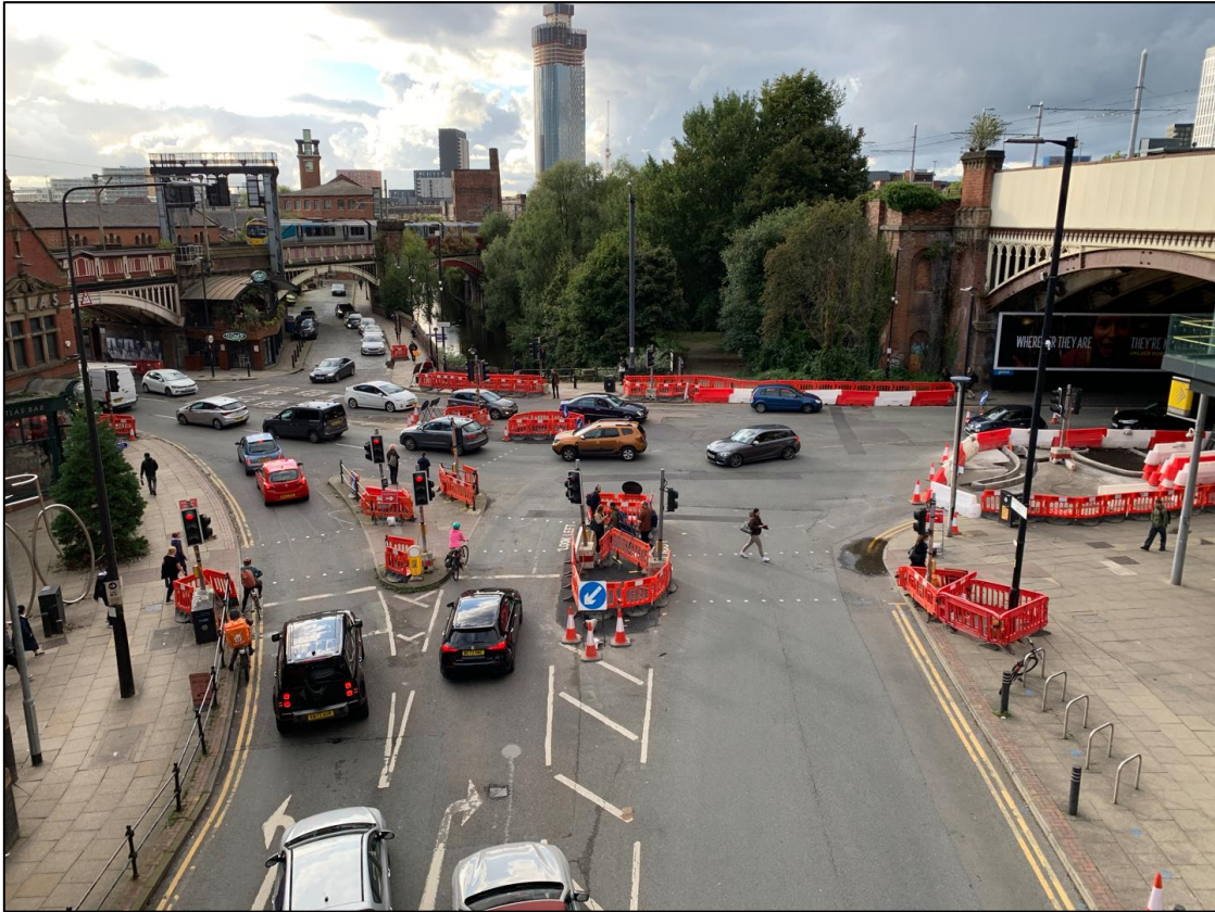
Figure 2.3 – West Facing View of Whitworth Street West / Deansgate / Castle Street / Bridgewater Viaduct Junction
