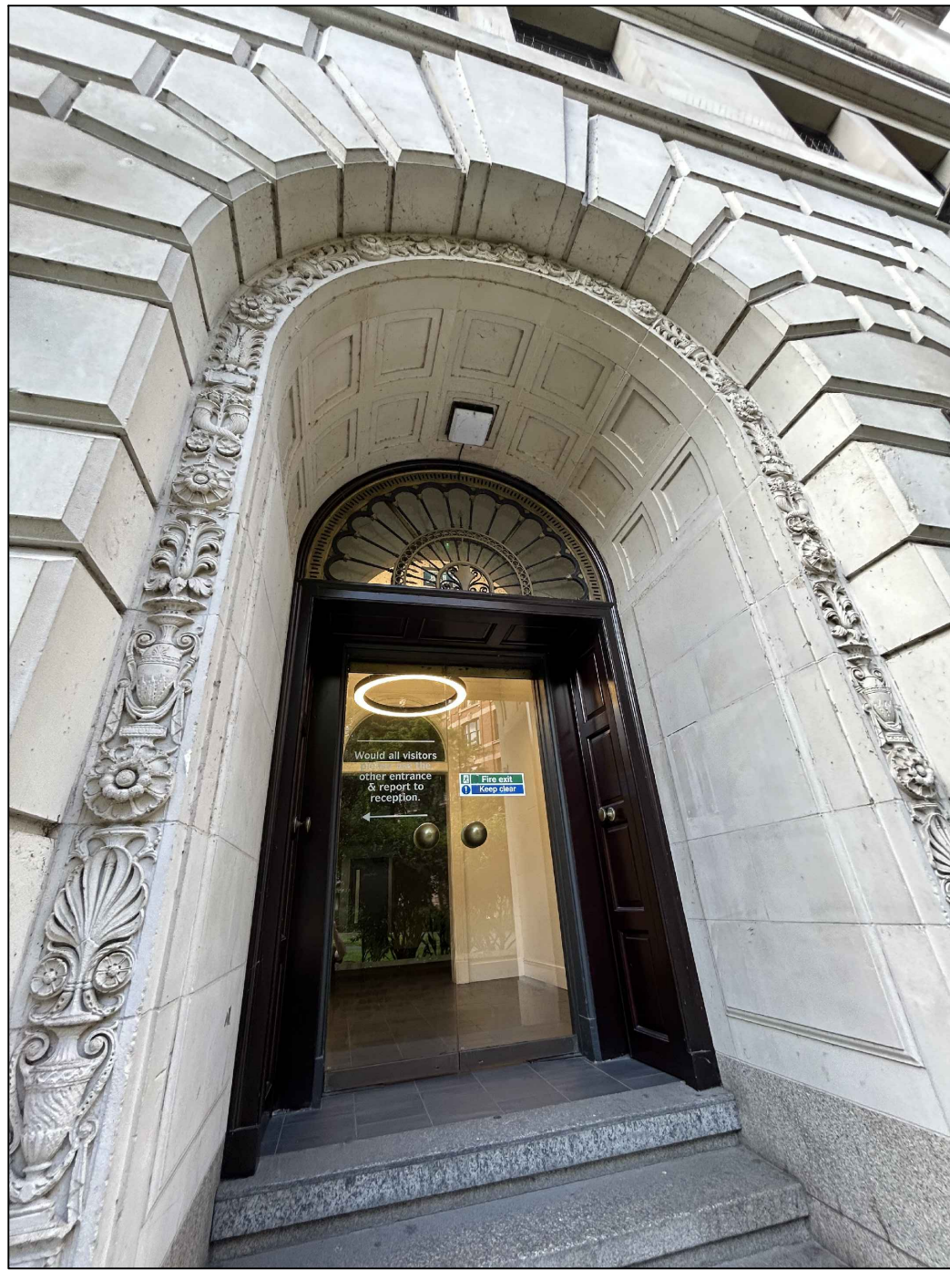
IMAGE OF EXISTING GLASS FIRE ESCAPE DOORS TO BE REPLACED AS PART OF PROPOSED WORKS
