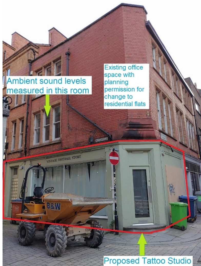
Figure 1.1. Photo of the existing retail shop where the proposed Tattoo Studio will be located. The internal ambient sound level measurement location inside a first floor room is also indicated.
