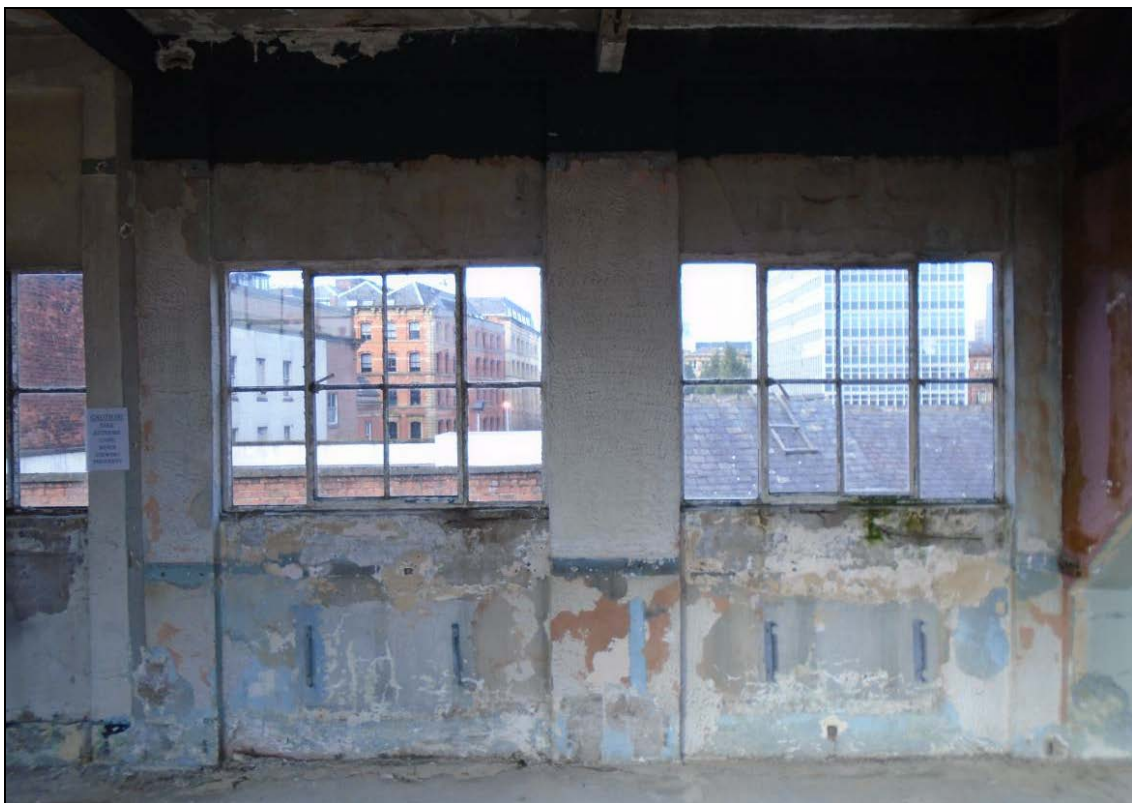
Plate 14: View of the rear sloping roof lights on the first floor
