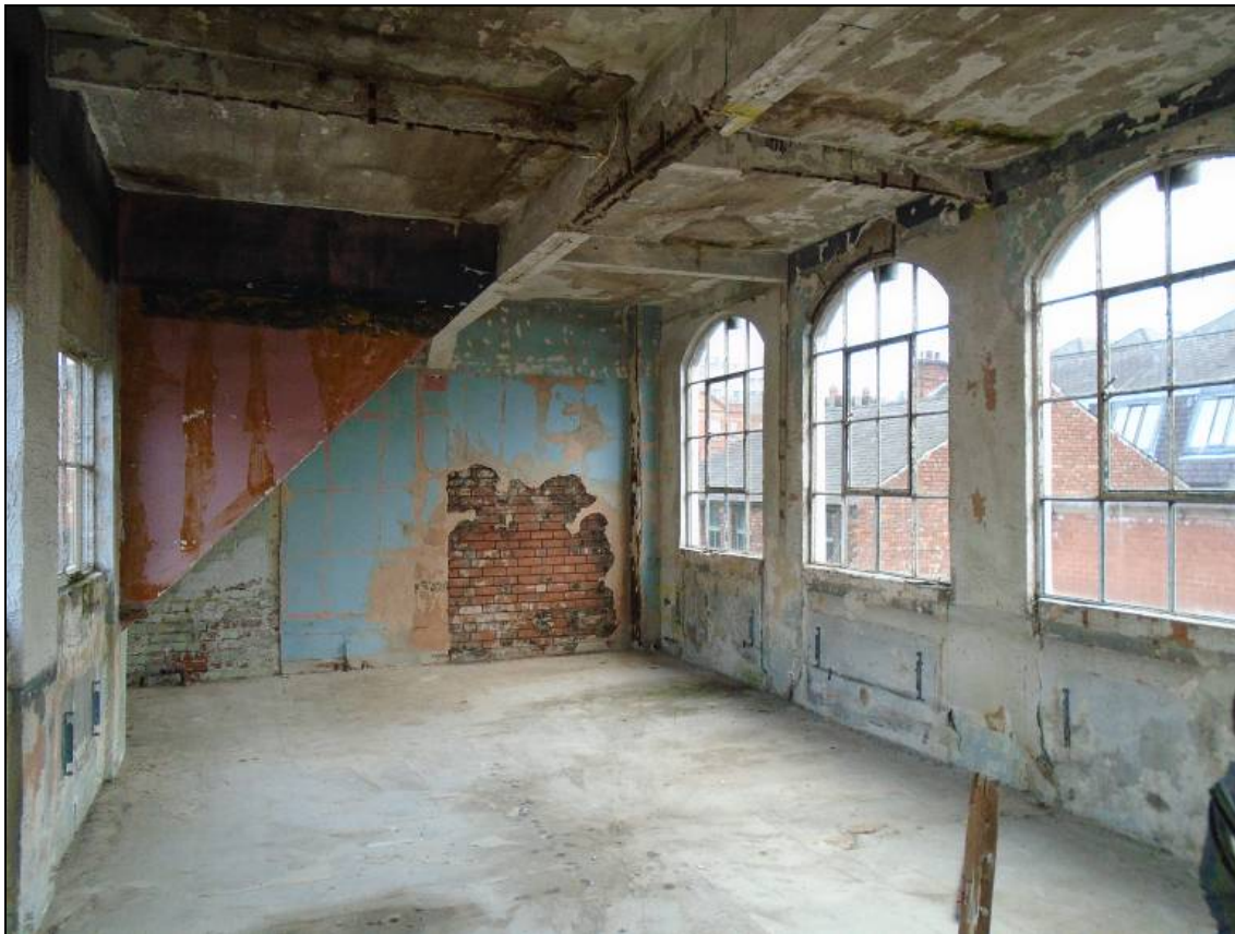
Plate 13: View of the rear sloping roof lights on the first floor
