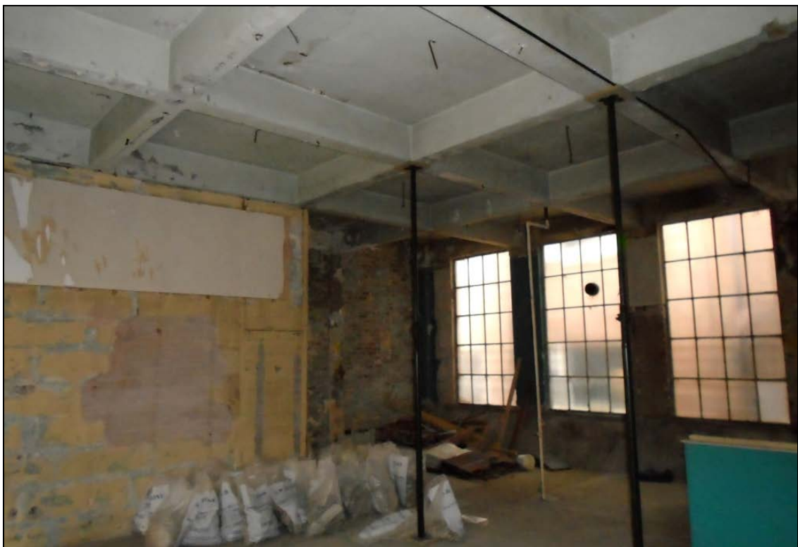
Plate 10: View of the rear windows on the ground floor, with original stairwell to upper floors to the left
