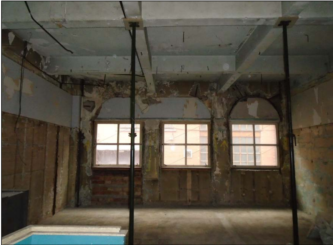
Plate 9: View across the ground floor, showing the windows in the front façade and the top of the inserted stair to the basement (painted blue)
