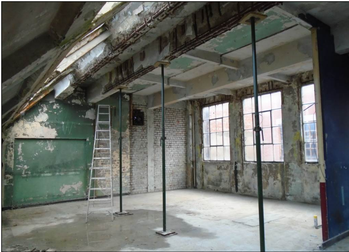
Plate 11: View of the front windows on the first floor, with stairwell to the left
