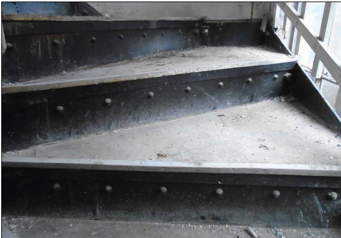
Plate 17: The metal stair frame and risers
