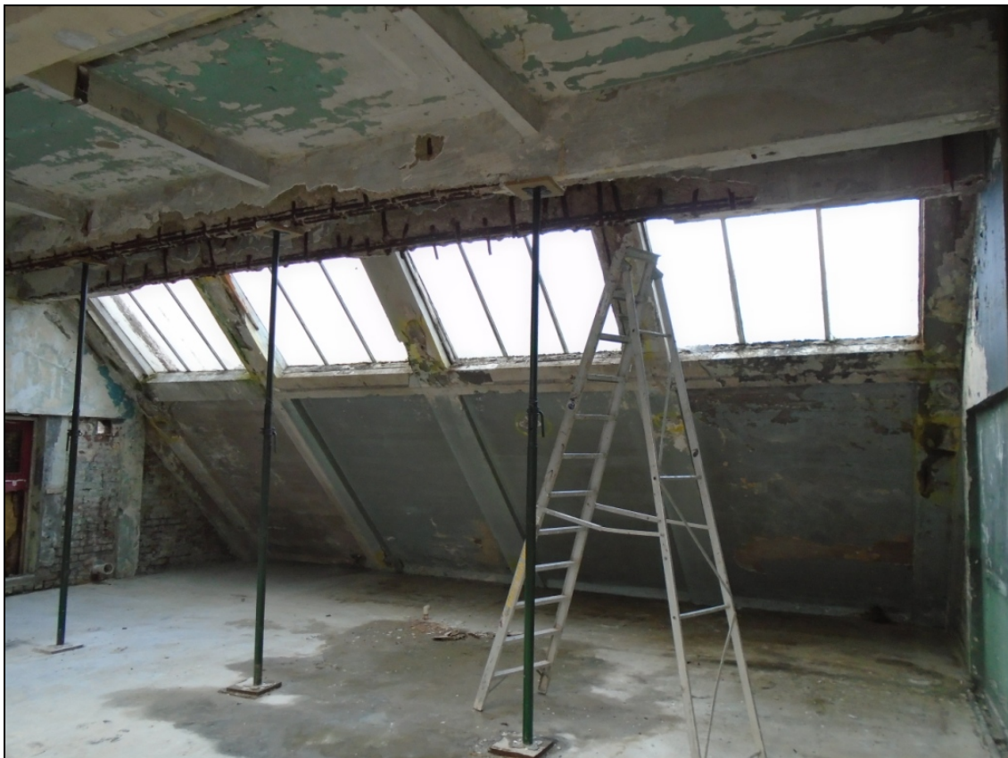
Plate 12: View of the rear sloping roof lights on the first floor
