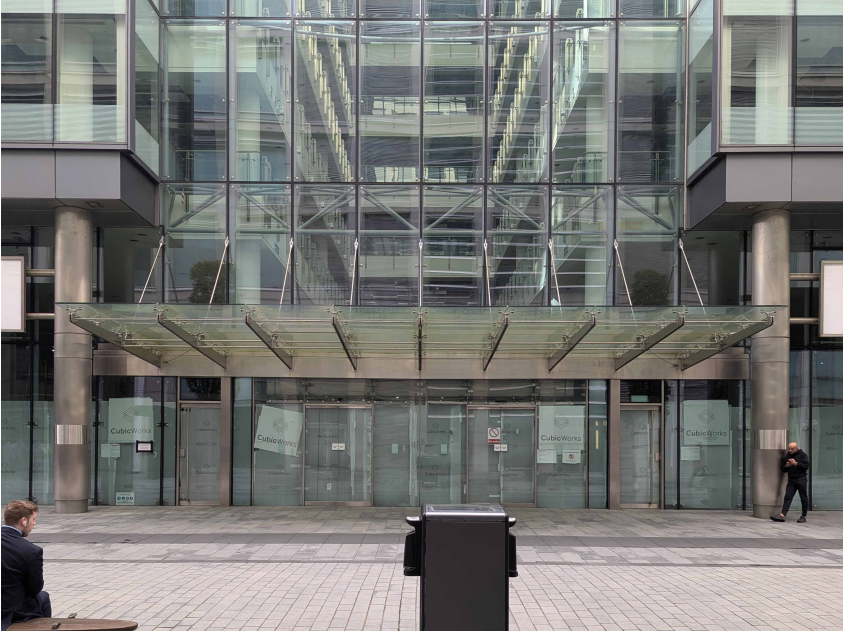
Photo of main entrance as existing
