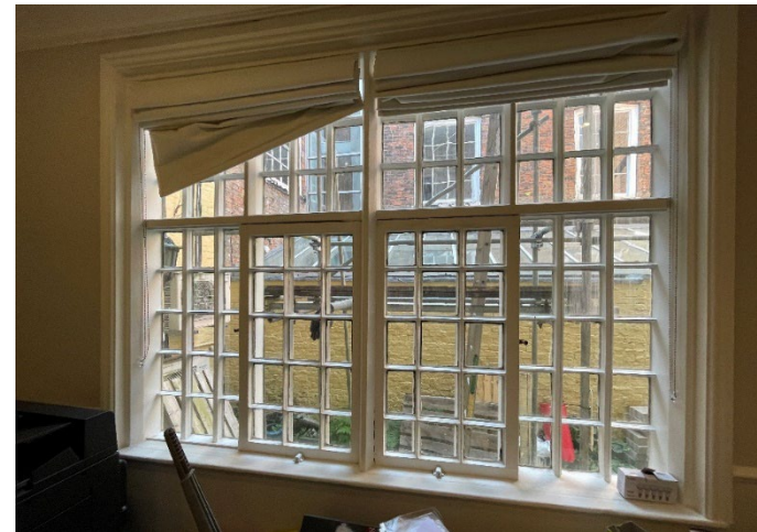
Plate 18: The interior of the ground-floor window to yard.
