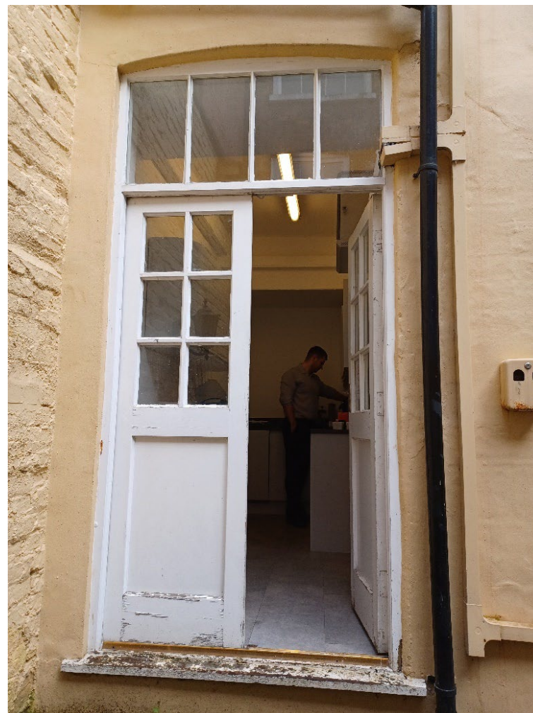
Plate 20: The external view of the door and over-light.
