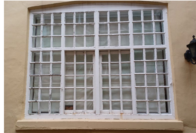
Plate 17: The exterior of the ground-floor window to yard.
