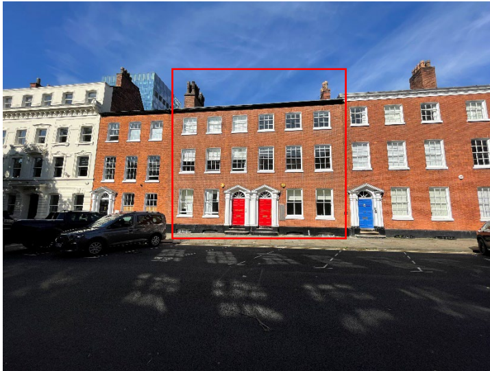
Plate 12: The Grade II Listed Nos. 18 & 20 St John Street.
