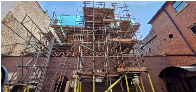
Plate 13: The rear elevation but obscured by scaffolding.
