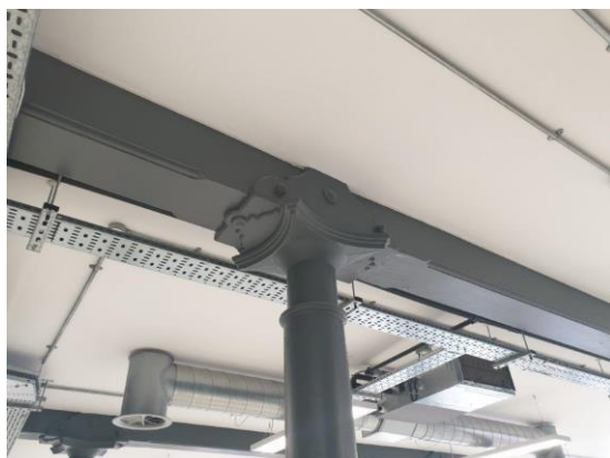
Image 3.1: Refurbished column head and beam detail
