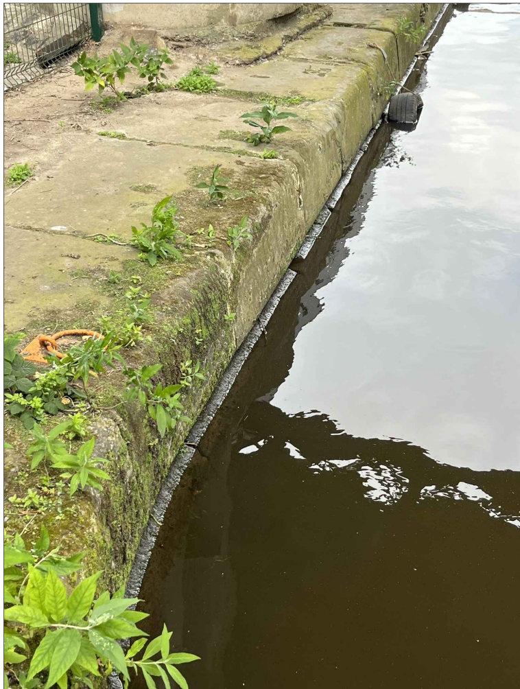
EXISTING NATURAL STONE COPINGS TO CANAL EDGE
