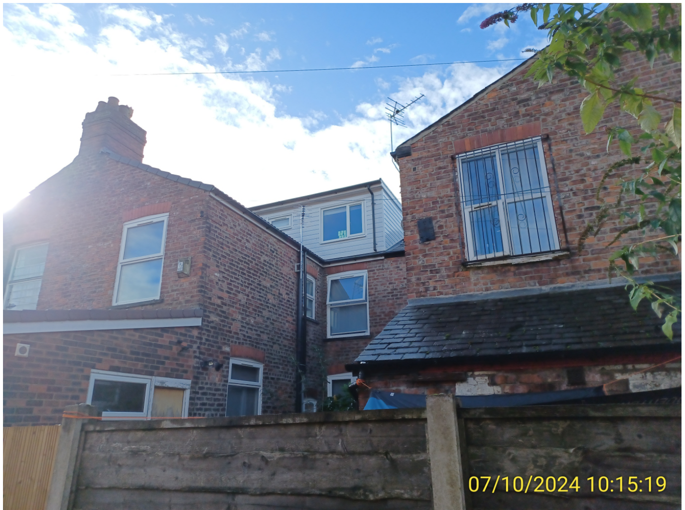
Photograph 1 White Clad Dormer as built at the application site. Source: Case Officer Site Visit Photographs
