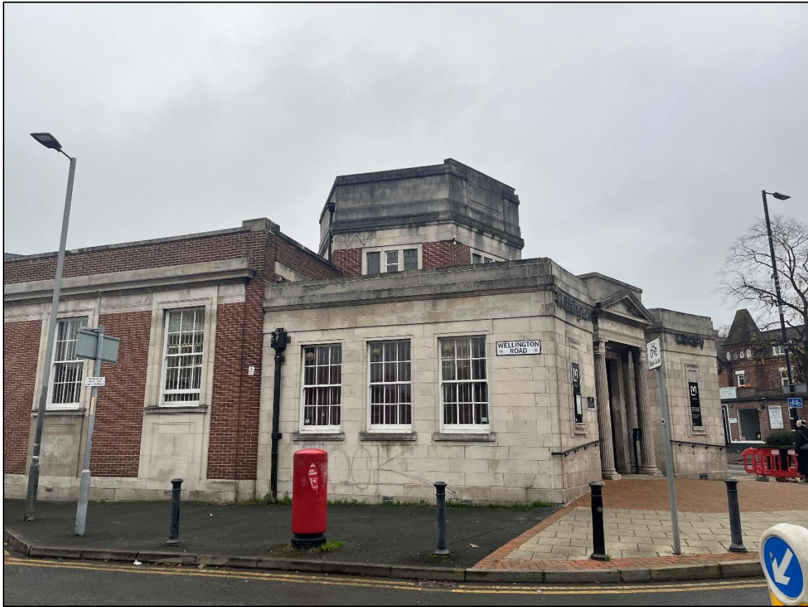
Plate 1 – Withington Library as seen from the west
