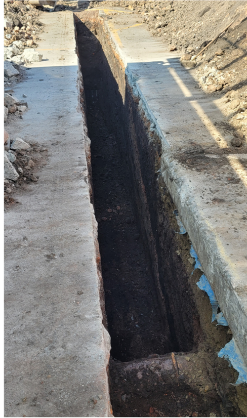
Photograph 3 – Trial Pit Viewing West
