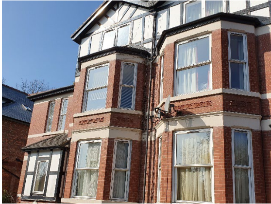
Photo 7: Bay windows with sandstone detailing.
