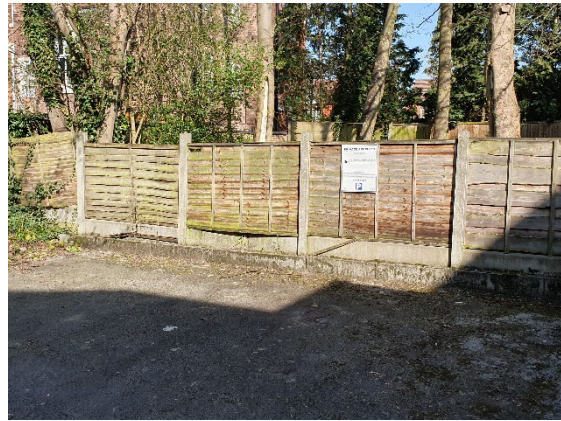
Photo 14: RHS timber panel and concrete post fence.
