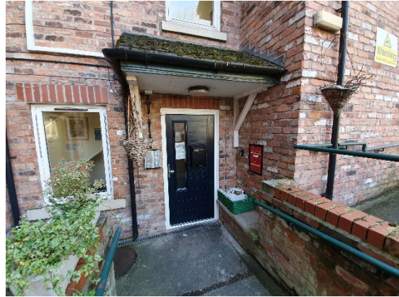
Photo 26: Main entrance door at rear.
