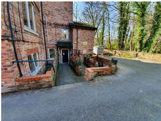
Photo 21: Main building access to rear.
