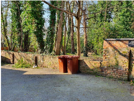
Photo 15: Rear brickwork garden wall.
