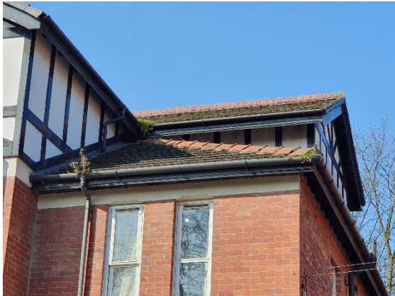
Photo 3: Interlocking concrete tiles to high level roofs.
