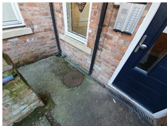
Photo 24: Drainage near main entrance door.
