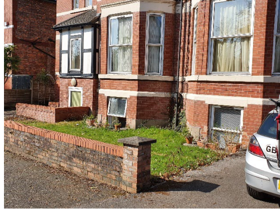
Photo 8: Low-level wall to site boundary.
