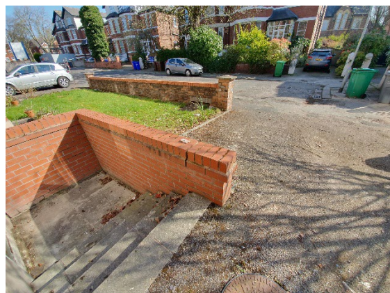
Photo 18: Low-level brick wall to front elevation.
