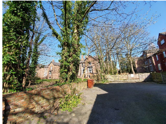
Photo 16: Rear brickwork garden wall.
