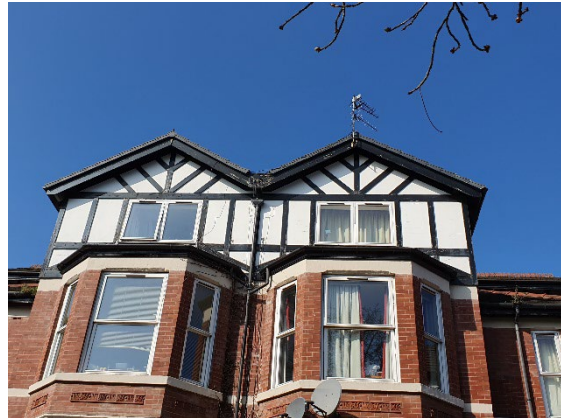
Photo 4: Mock Tudor to third floor.
