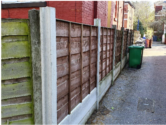
Photo 13: RHS timber panel and concrete post fence.
