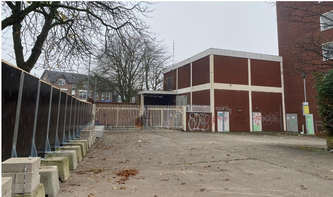
View of existing hoarding and kentledges placed as support according to the blue line arrangement (Figure 1) along the northern border of the site (facing east). Trees in G4 shown in the right side of image.
