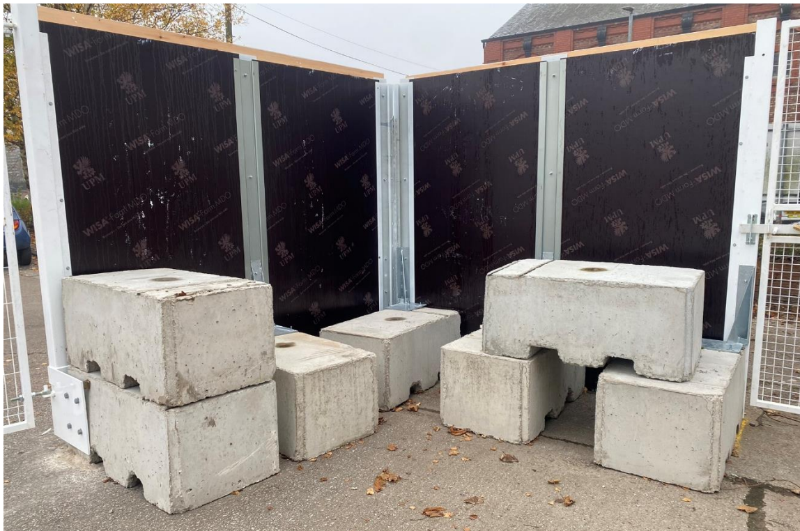
View of existing hoarding and kentledges placed as support according to the blue line arrangement (Figure 1) in the north-western corner (facing north). Gate to the left side of image represents main access point into the demolition area (positioned north-west relative to G4).
