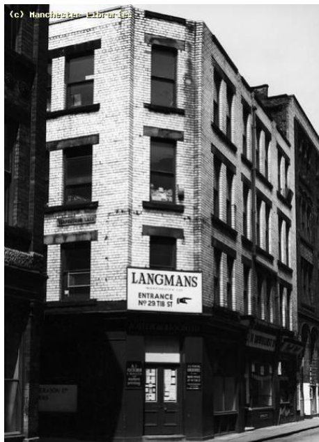
Figure 3 - 25 Tib Street (previously 34) photographed in 1959 (Source: Source Manchester Archives)
