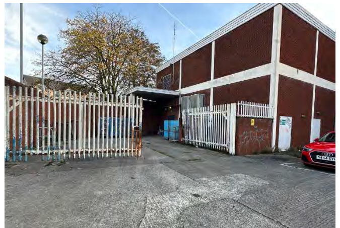
4. Refuse area in north of site behind Graeme House.
