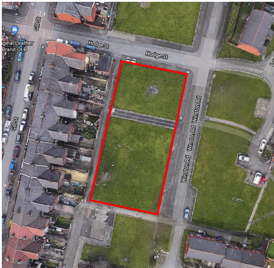
Figure 1.1 – Aerial view of existing site
