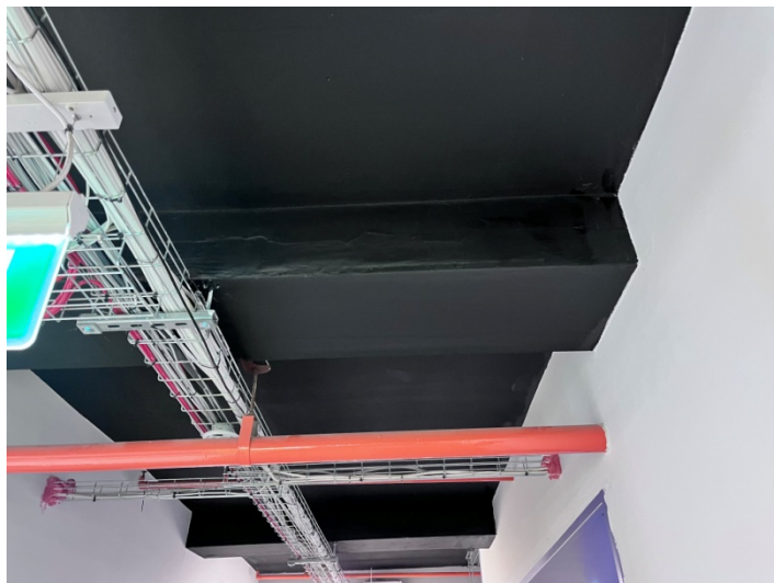
Image of existing ceiling with electrics within cable trays and sprinkler system pipework.
