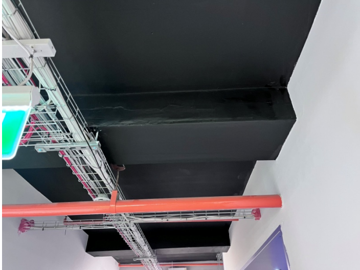
Photograph of ceiling
