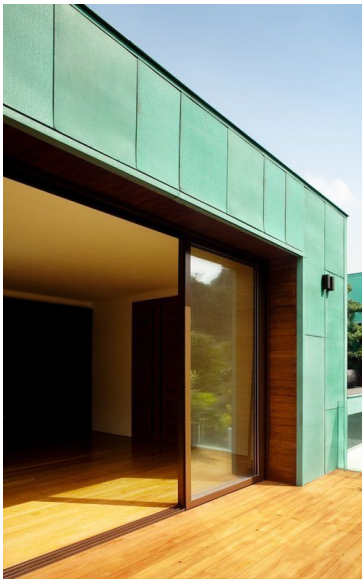
Façade with copper metal cladding
