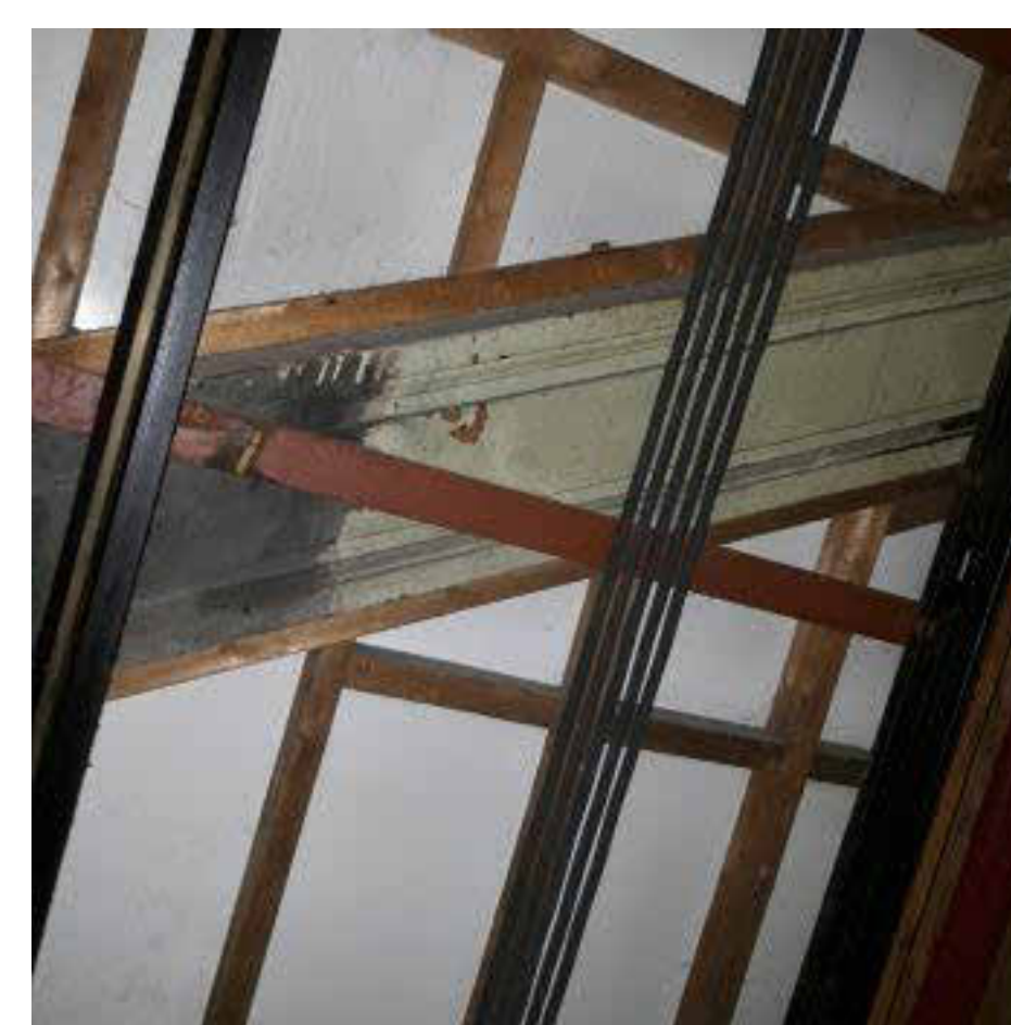
Internal shaft view of cast iron stringer
