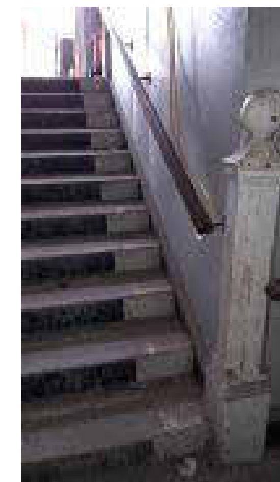
Existing concrete treads and cast iron newel post. Handrail and shaft to be removed
