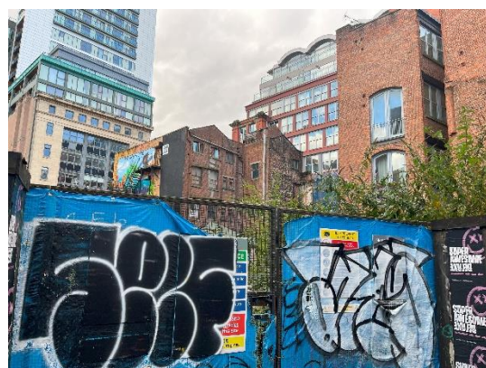
Figure 2.3 The site as seen from the rear near the Abel Heywood public house.
