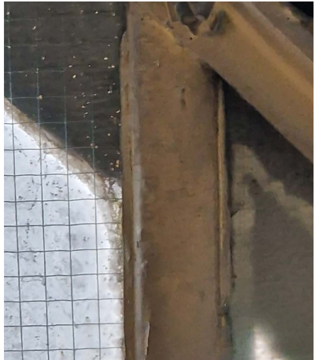
Figure 2 Glazing Bar, Internal Photograph
