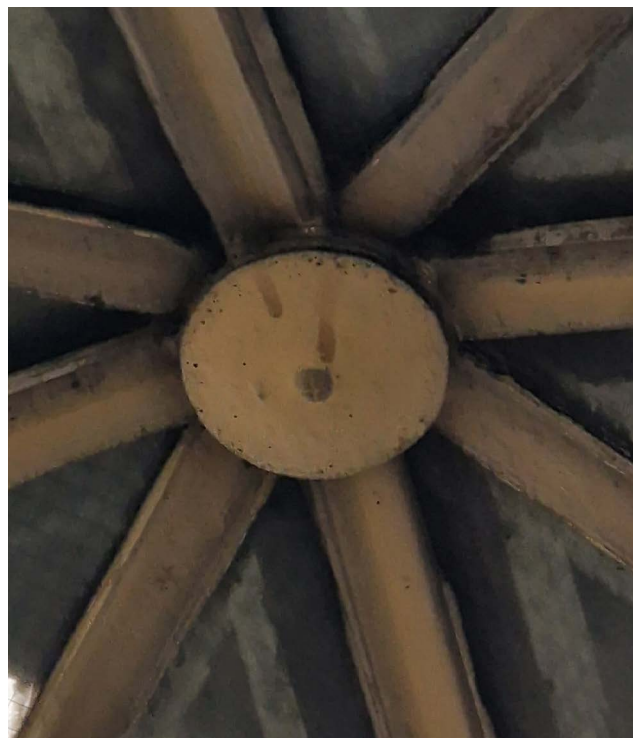
Figure 4 Cental Boss, Internal Photograph
