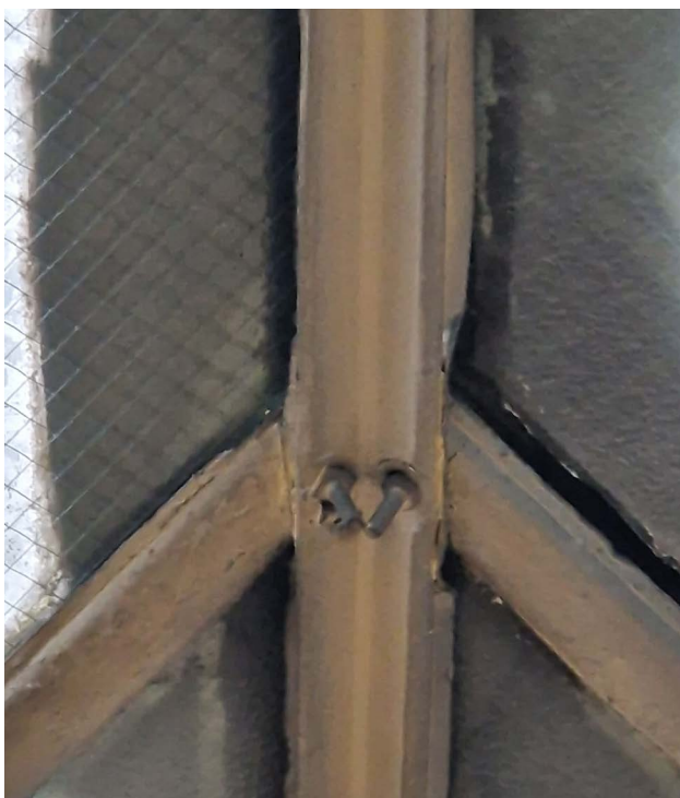
Figure 3 Hip Section, Internal Photograph
