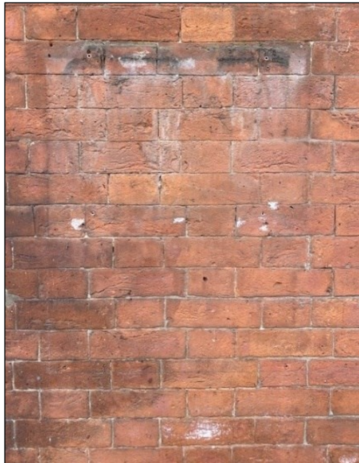
Existing Picture – Bellhouse Façade
