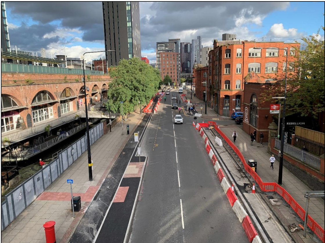
Figure 3.4 – East Facing View of Whitworth Street West
