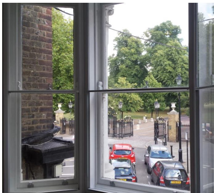
Example of the proposed white aluminium SGS for traditional vertical sliding sash windows. Sash windows with existing/restored shutters to omit secondary glazing or have slim profile vertical sash SGS or 'click out units'/frames of similar design [see*]
