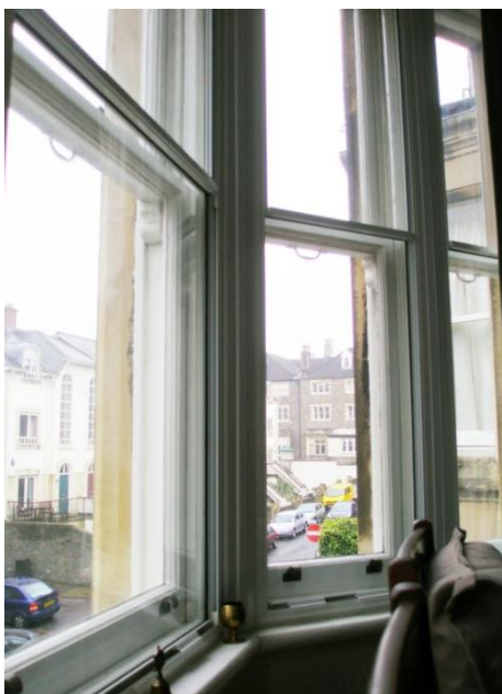
Example of the proposed white aluminium secondary glazing system [SGS] for traditional vertical sliding sash windows with sliding secondary sashes mimicking the pattern of the outer window to be used at Fenton House.
