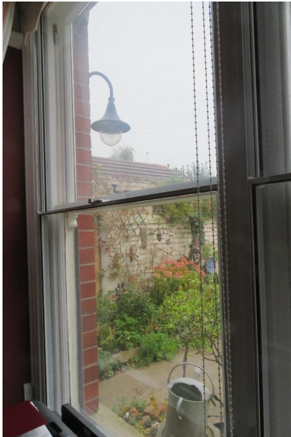
Details of slim profile SGS meeting rail with a one over one pane traditional sash window behind, and SGS at the internal window sill.
