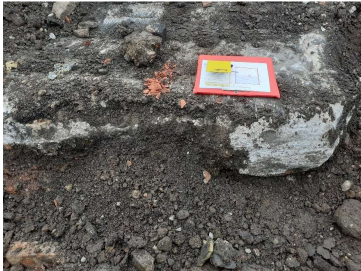
Plate 14: Friday 25 th August 2022. Asbestos hotspot 3 – image of the northern side.
