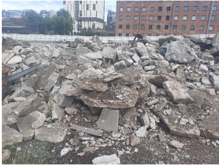
Plate 32: Monday 5 th September 2022. Concrete which was broken out on site.
