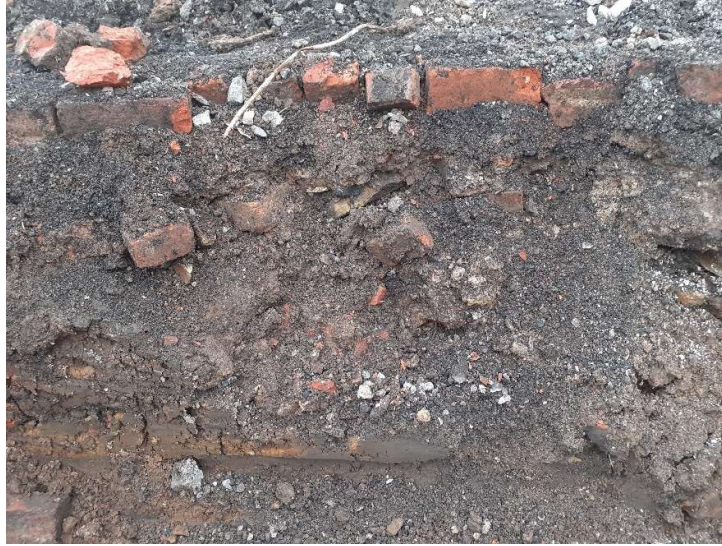
Plate 9: Friday 25 th August 2022. Asbestos hotspot 2 – image of the northern side.
