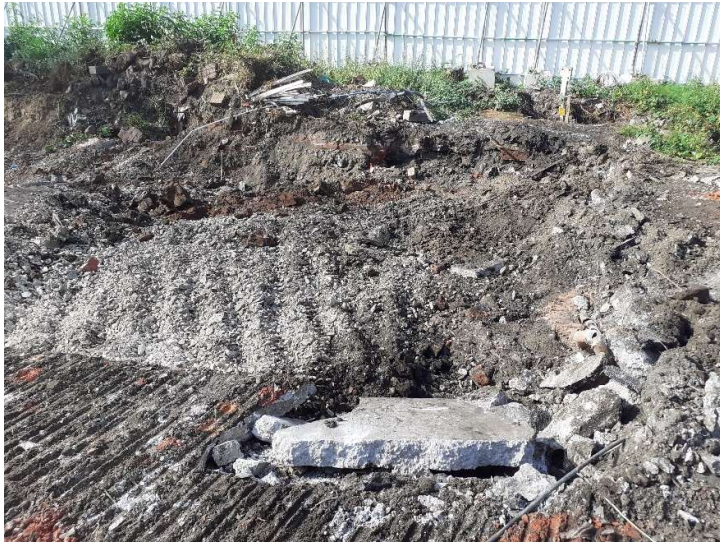
Plate 28: Monday 5 th September 2022. Demolition and excavation debris on site.
