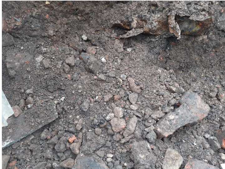
Plate 3: Friday 25 th August 2022. Asbestos hotspot 1 – image of the northern side.
