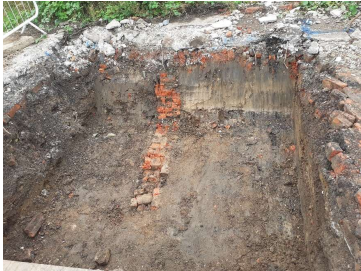
Plate 7: Friday 25 th August 2022. Asbestos hotspot 2 – overview of excavation.
