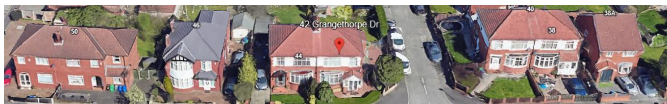
View of front-facing roof slopes along Grangethorpe Drive
